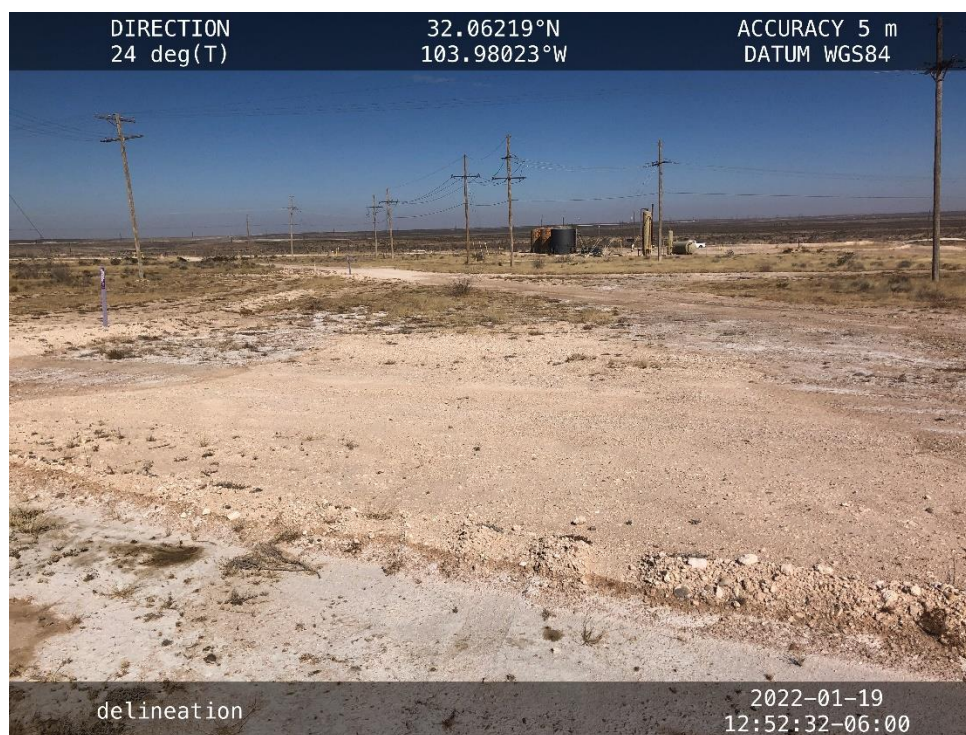
PHOTO 6: View of release in pipeline right-of-way.
