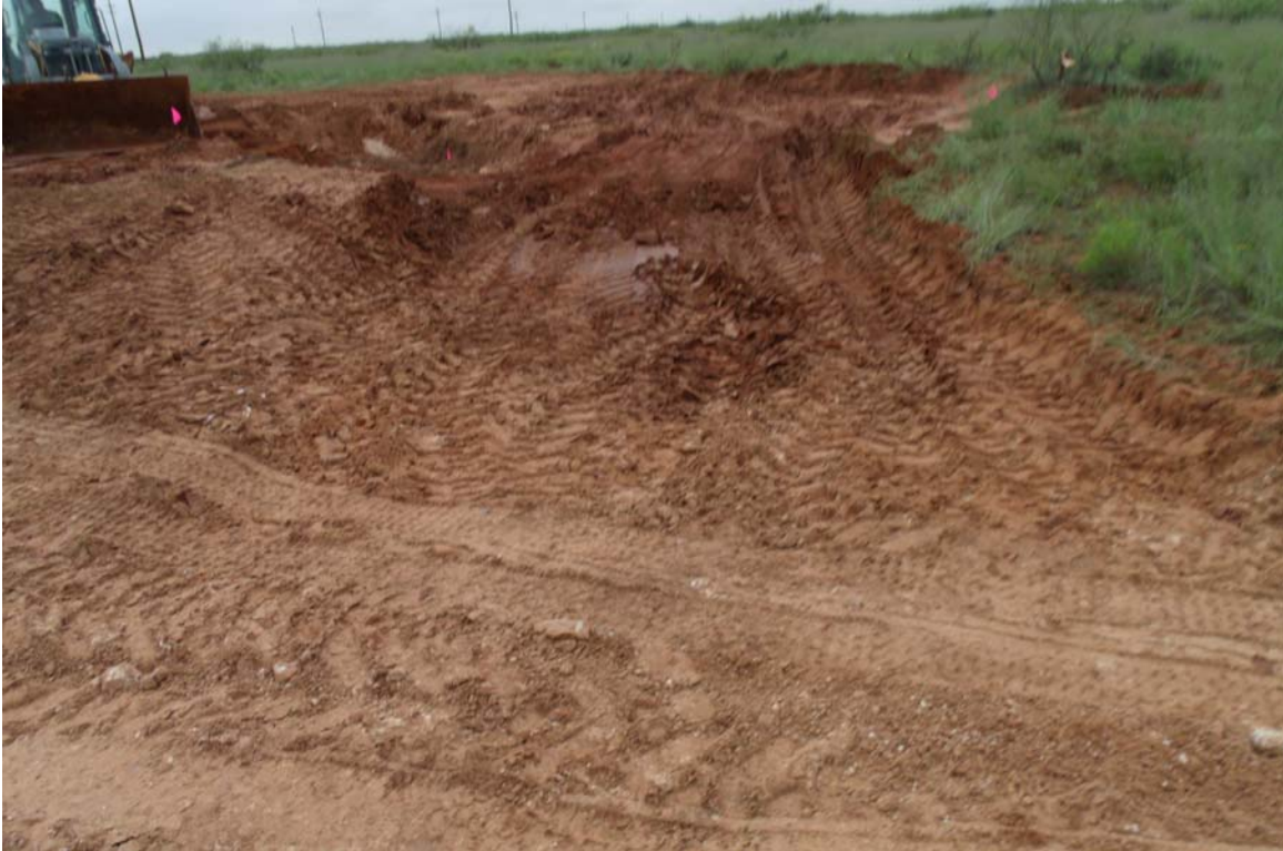
Photograph #9 – Excavated area
