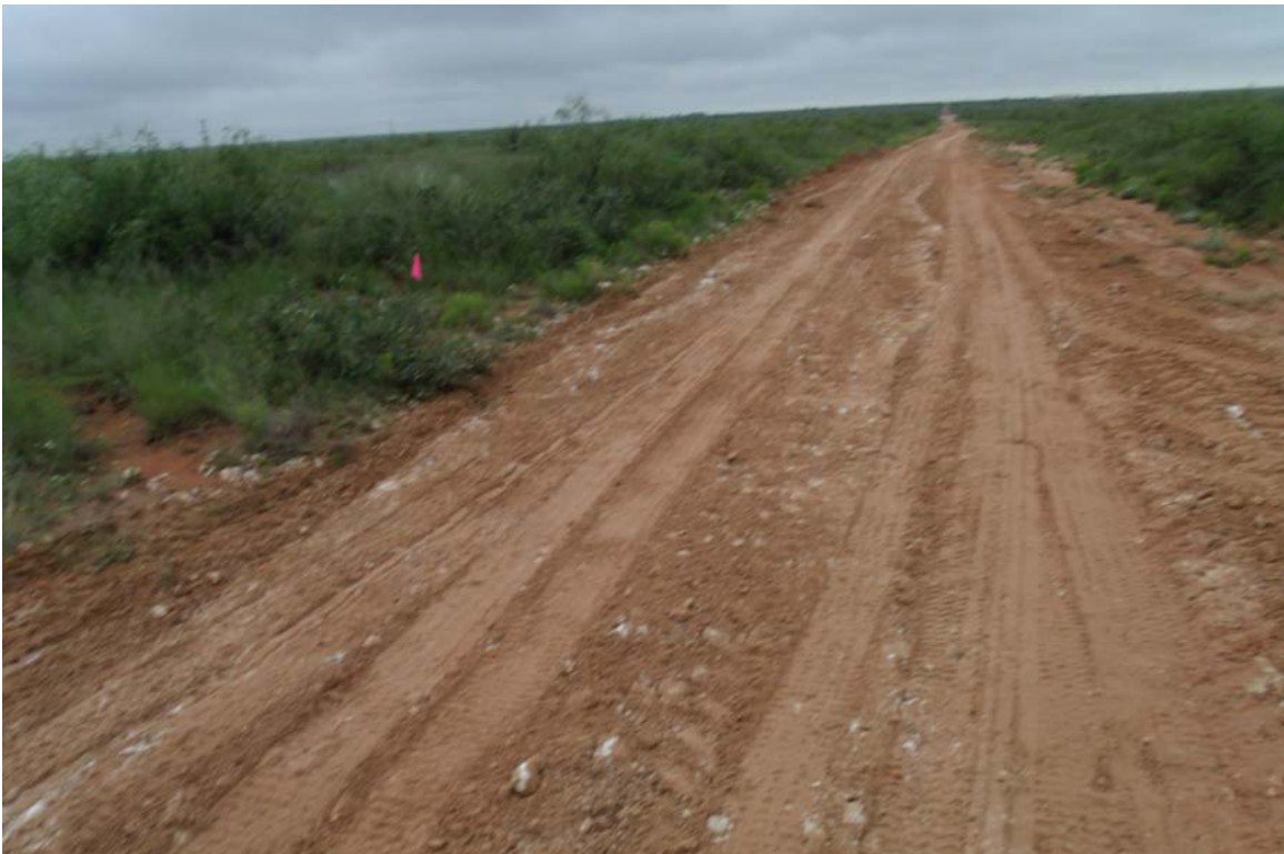
Photograph #10 – Excavated area
