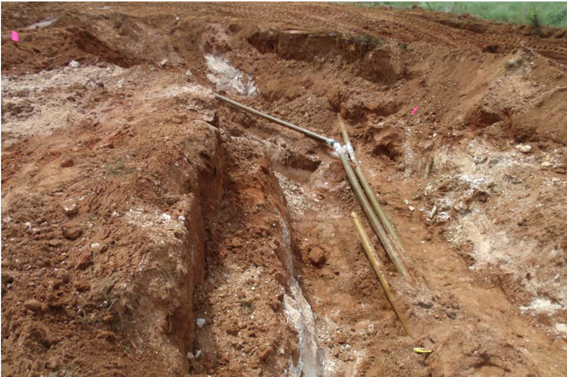
Photograph #8 – Excavated area
