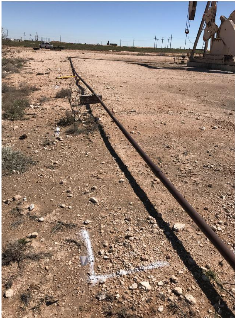
View of release area prior to excavation.
