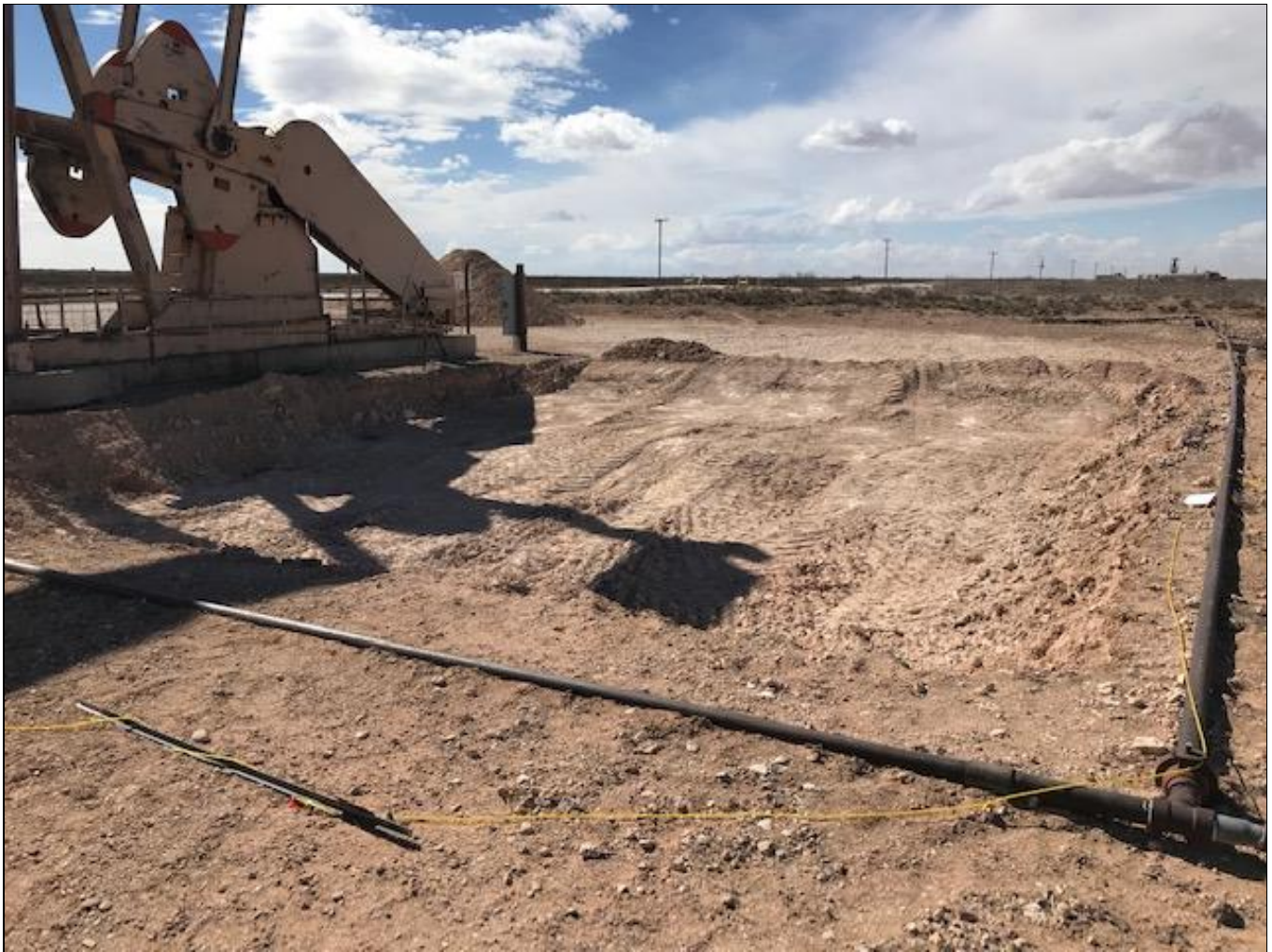
West facing view of the larger excavation.
