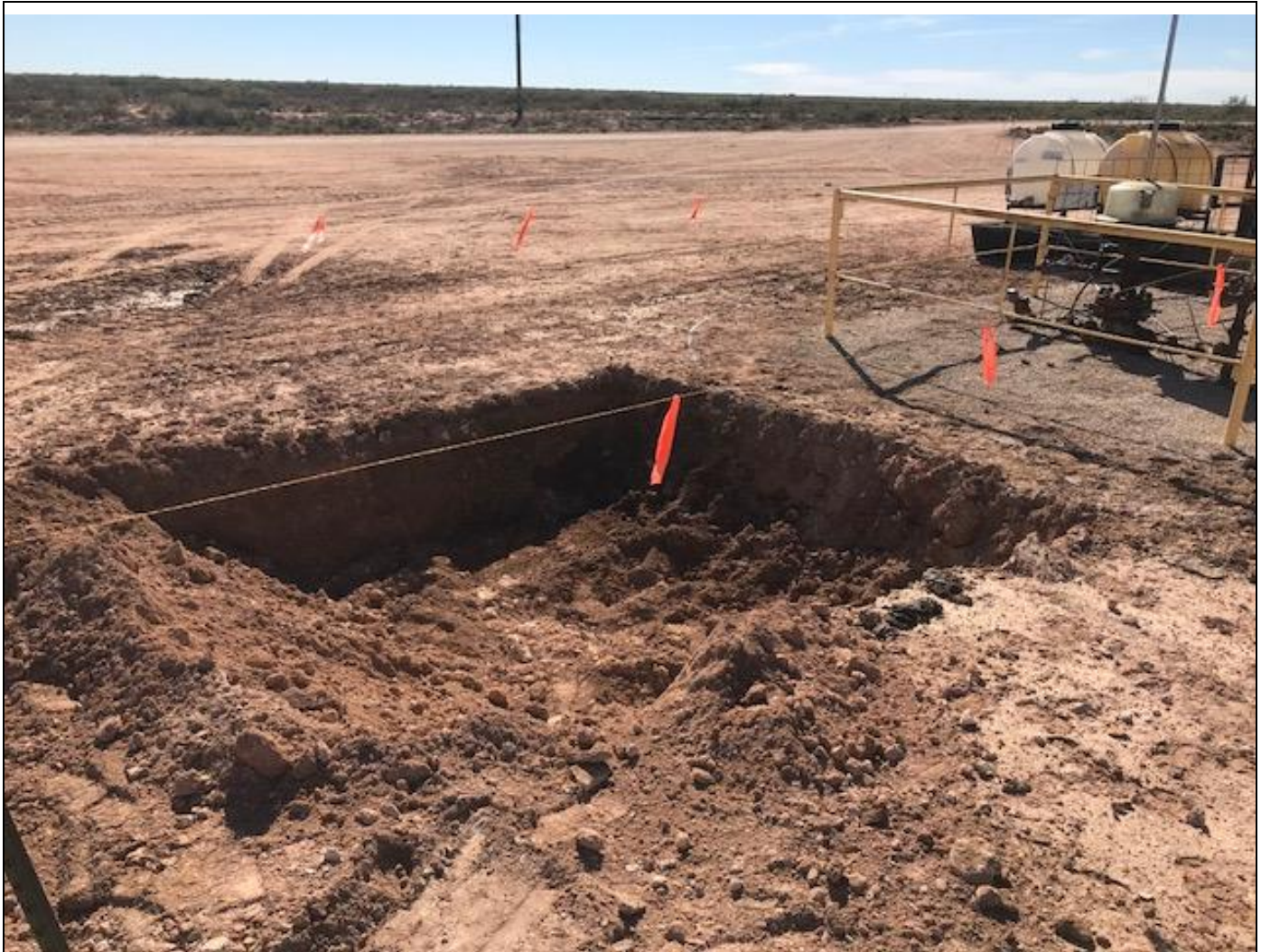
Southeast facing view of the smaller excavation.
