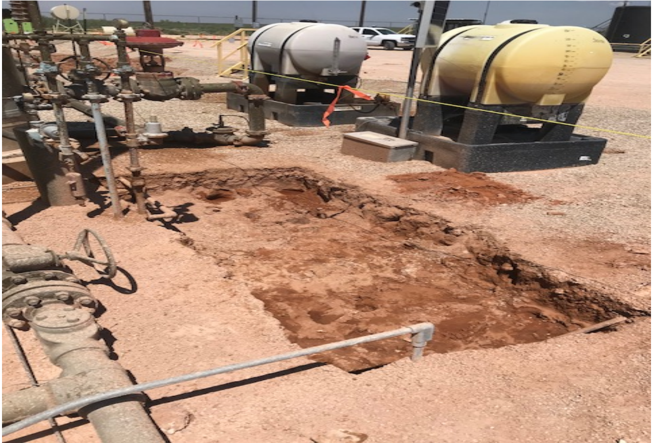
Northeast facing view of southern excavation.
