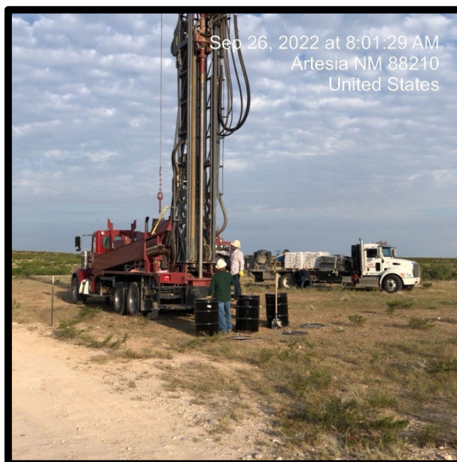
PHOTOGRAPH NO. 1 – A view of the soil boring/temporary well “SB-1” installation process. The view is towards the northwest.
