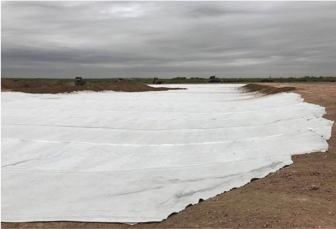
**Figure 9** - View of installation of the bentonliner, facing north.
