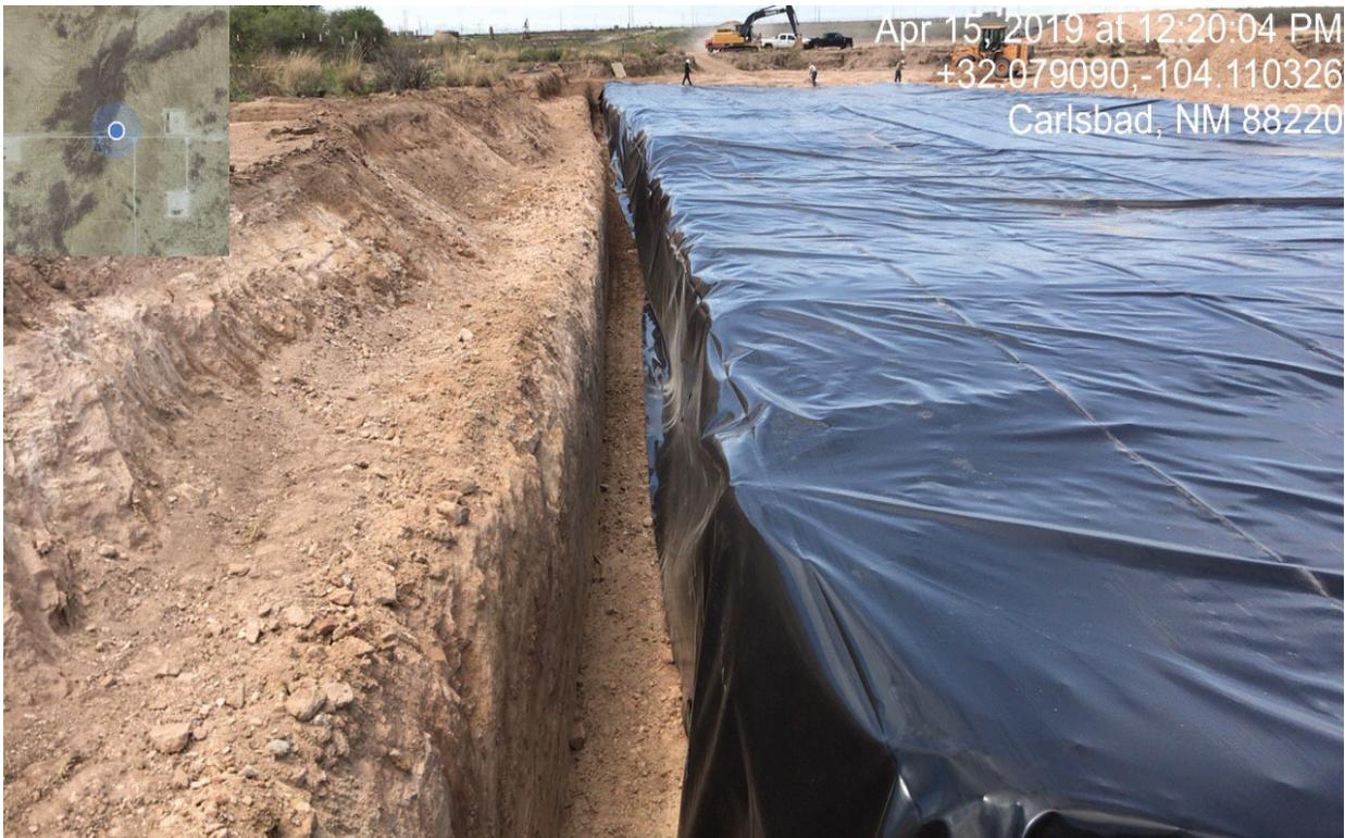
**Figure 4** - View of portion of the liner keyset, facing west.
