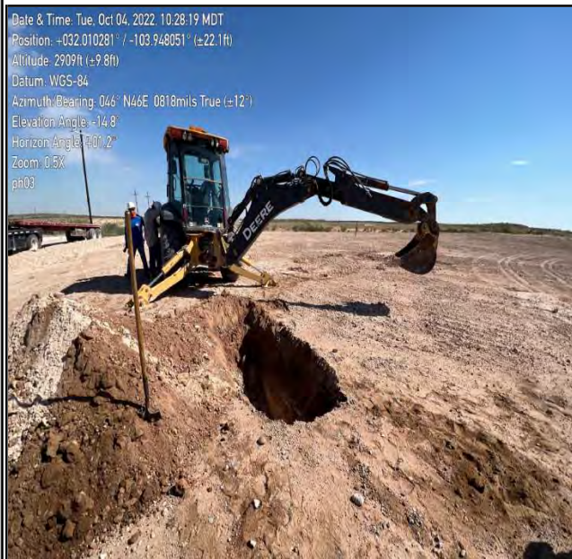
Photograph 3 Date: 10/04/2022 Description: Pothole Sampling (PH03) View: Facing West
