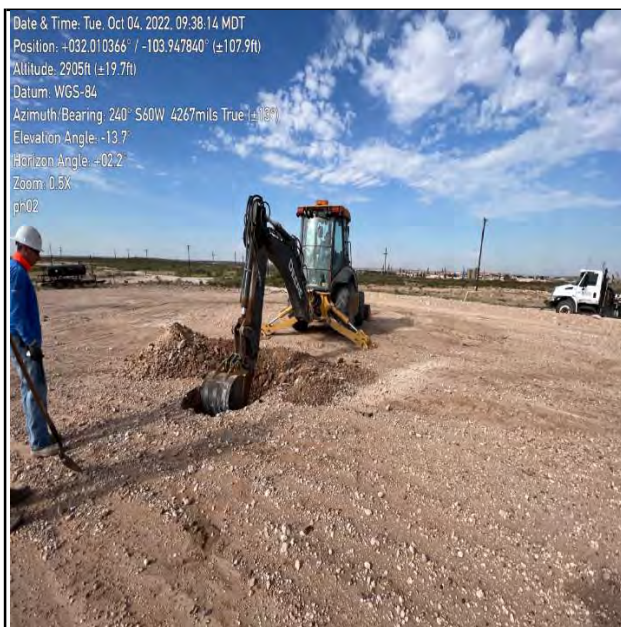
Photograph 2 Date: 10/04/2022 Description: Pothole Sampling (PH02) View: Facing West
