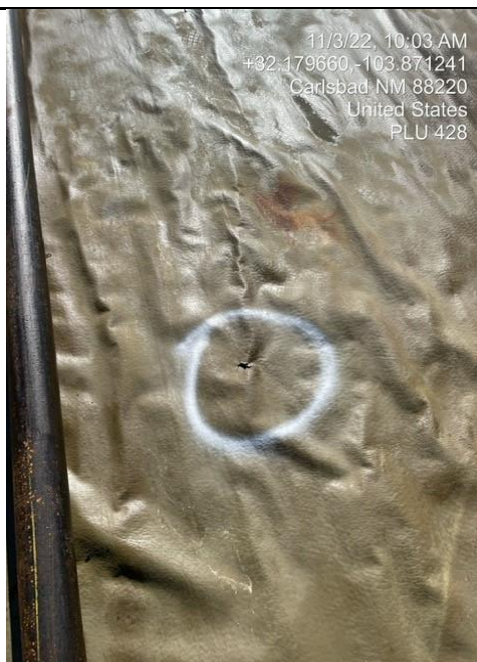
Photograph 2 Date: 11/03/2022 Description: Location of failing liner View: Southeast
