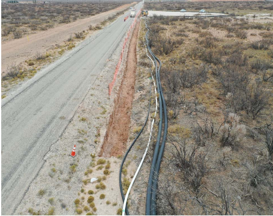
Excavation Activities, Facing South
