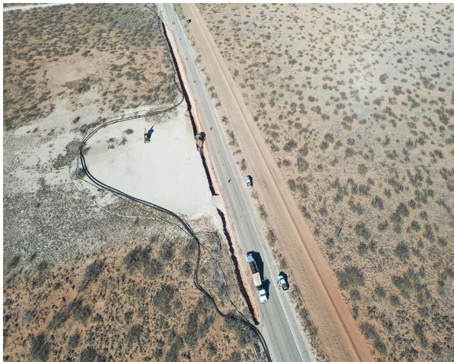
Aerial Overviews of Work Area, Facing North
