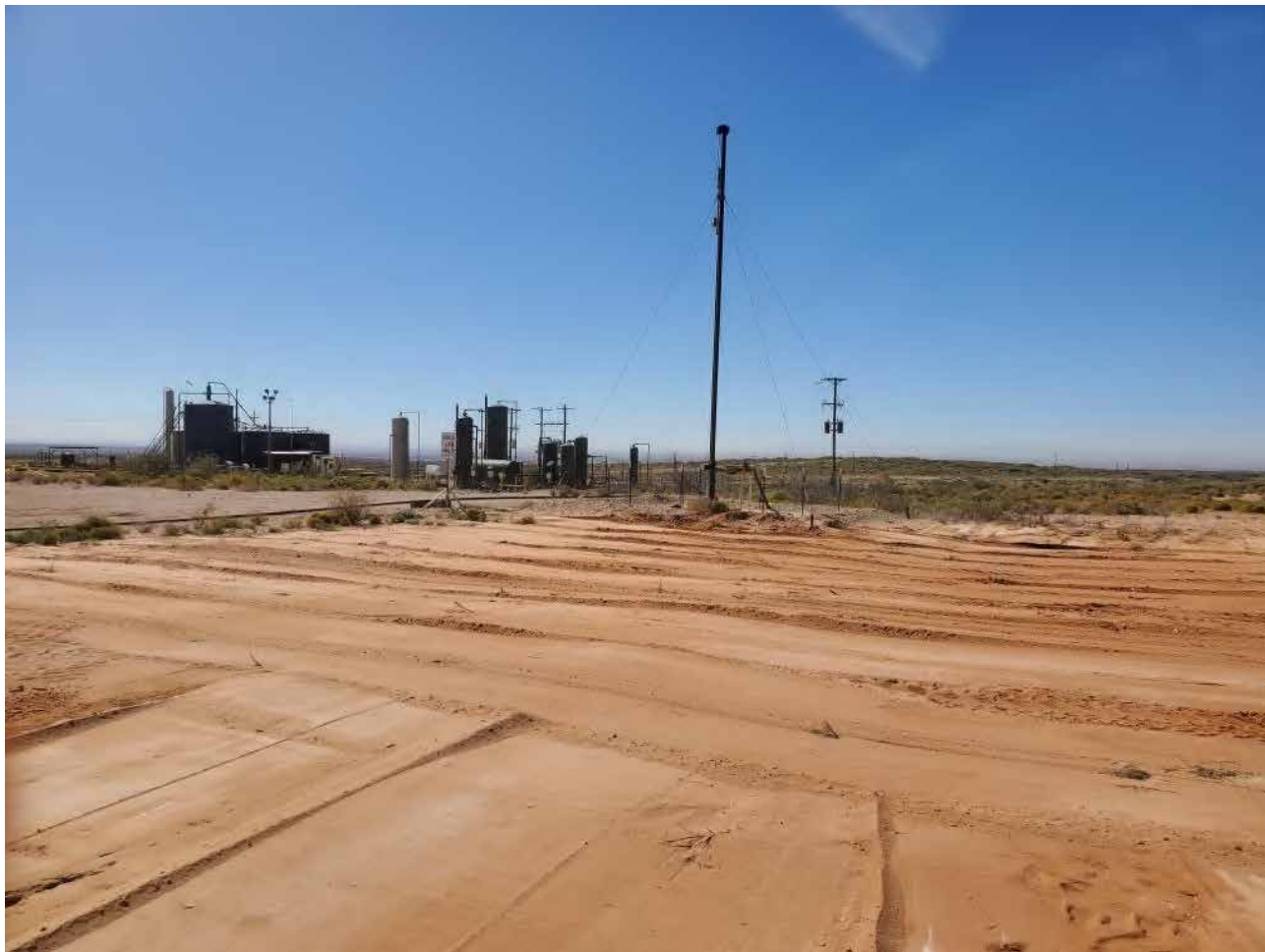
Backfilled/contoured excavation area (2RP-4396, 2RP-4397).
