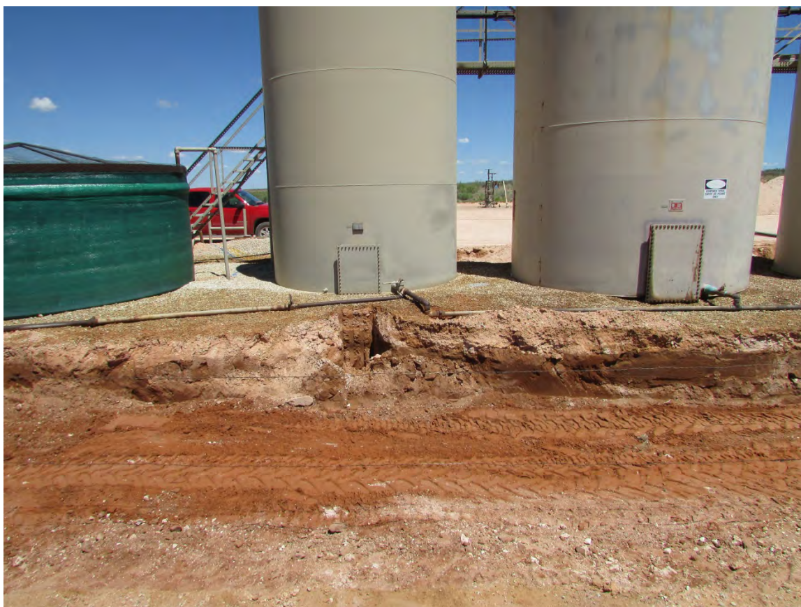
Middle of battery excavation facing North, August 18, 2016
