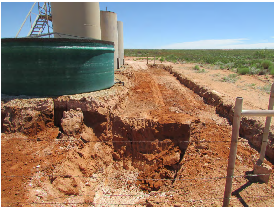
Southwest corner of battery excavation facing East, August 18, 2016
