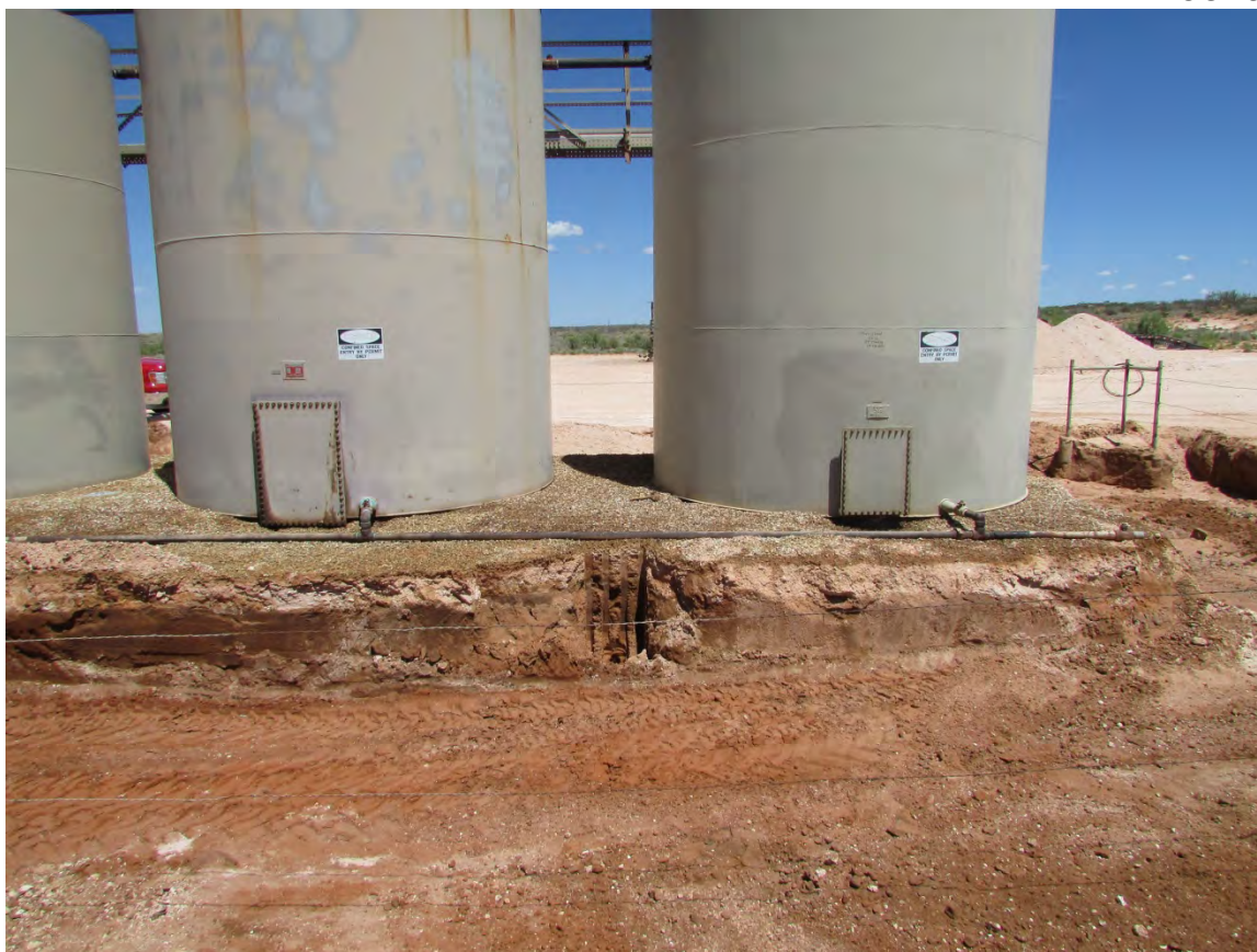
Middle of battery excavation facing North, August 18, 2016
