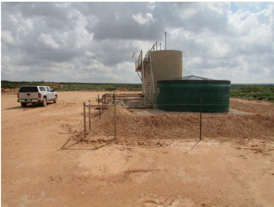
Northwest corner of backfilled tank battery and new firewall facing East, September 3, 2016
