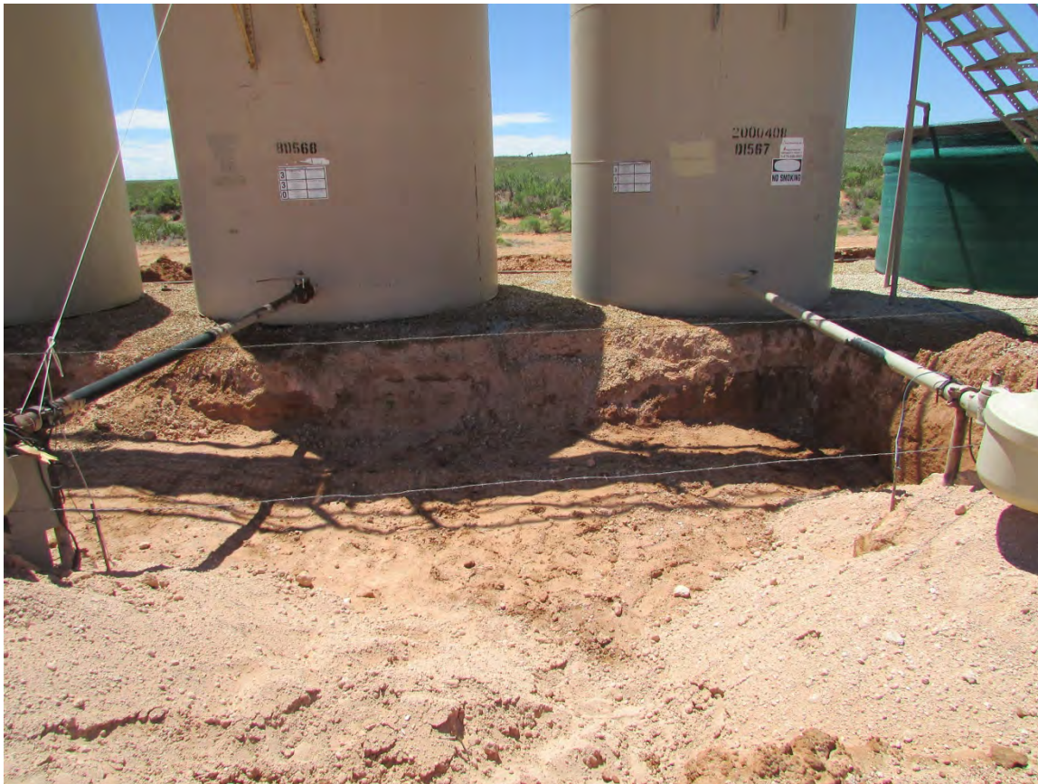
Middle of battery excavation facing South, August 18, 2016
