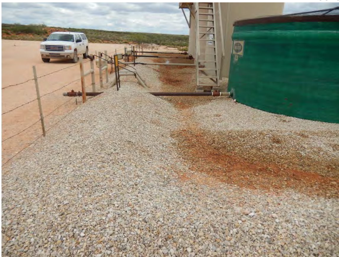
Stained Area inside firewall facing East, June 1, 2016
