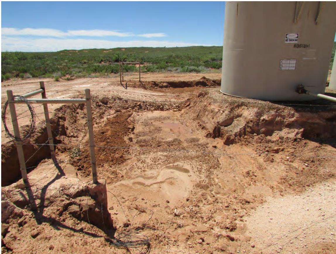
Northeast corner of battery excavation facing South, August 18, 2016
