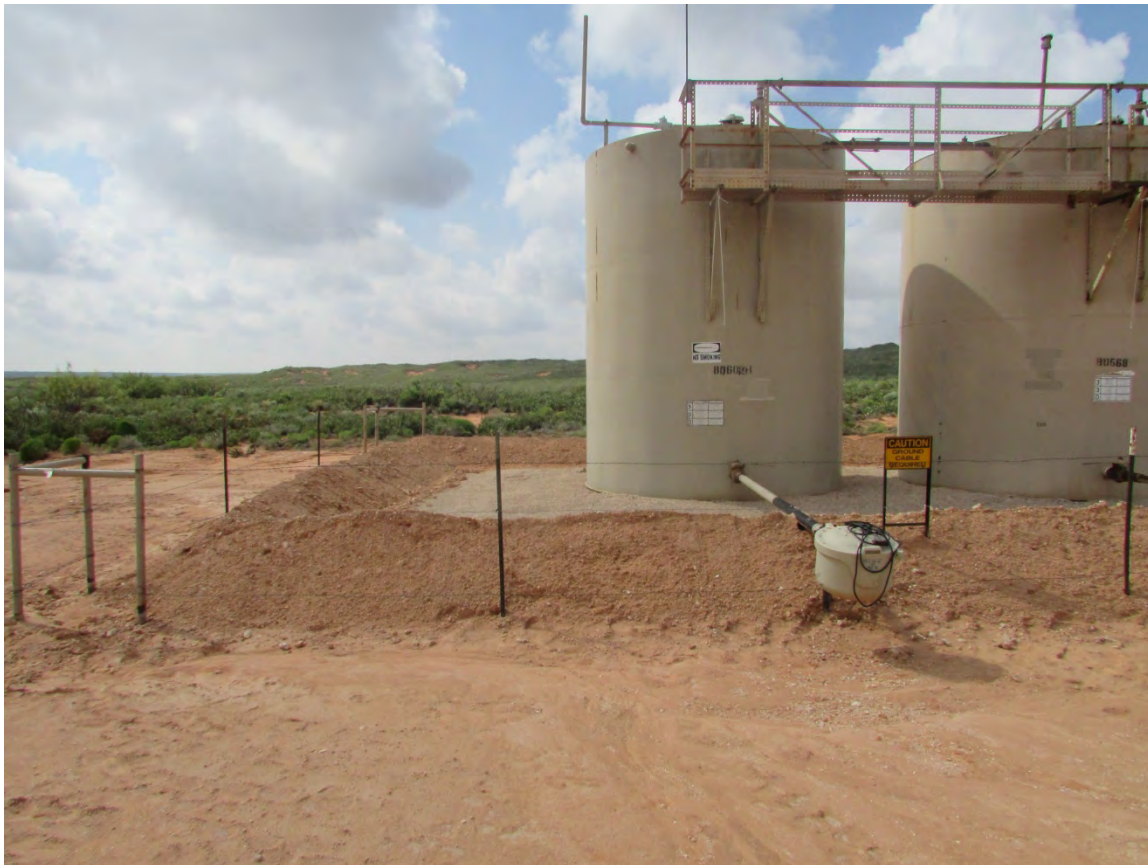
Northeast corner of backfilled tank battery and new firewall facing South, September 3, 2016
