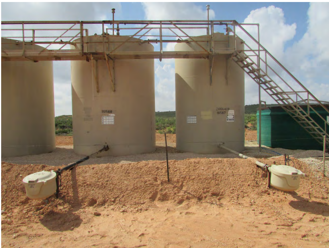
Middle of backfilled tank battery and new firewall facing South, September 3, 2016
