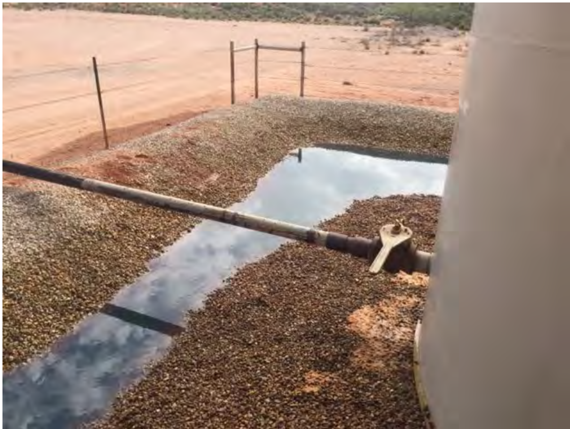
Crude Oil inside firewall near Northwest corner (DP-1) facing Northeast, May 20, 2016
