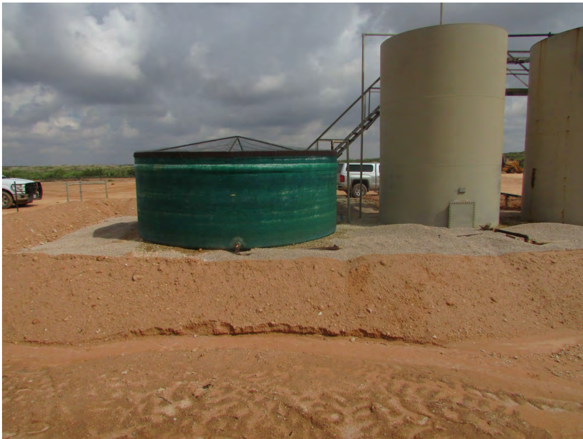
Southwest corner of backfilled tank battery and new firewall facing North, September 3, 2016
