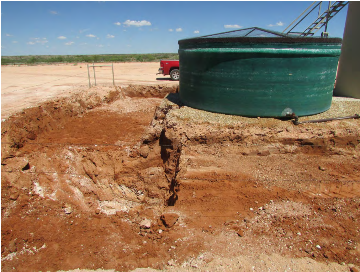
Southwest corner of excavation facing North, August 18, 2016
