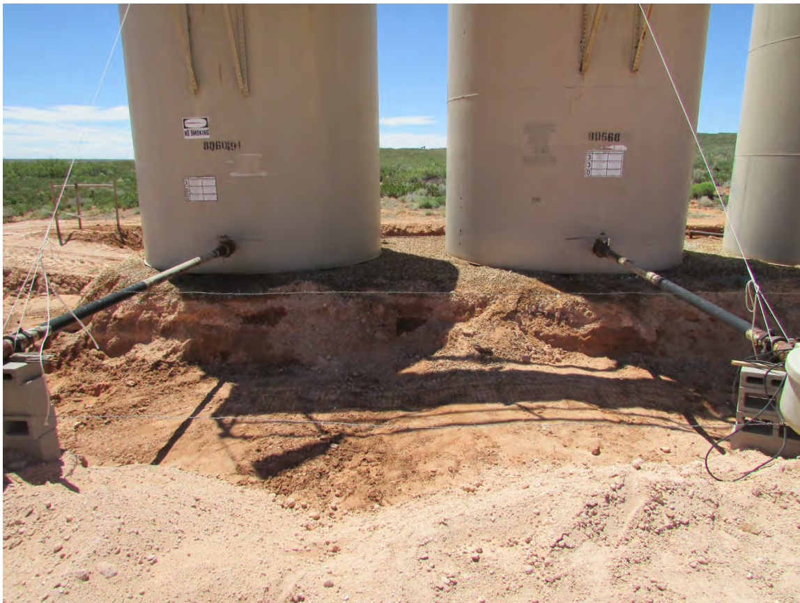
Middle of battery excavation facing South, August 18, 2016
