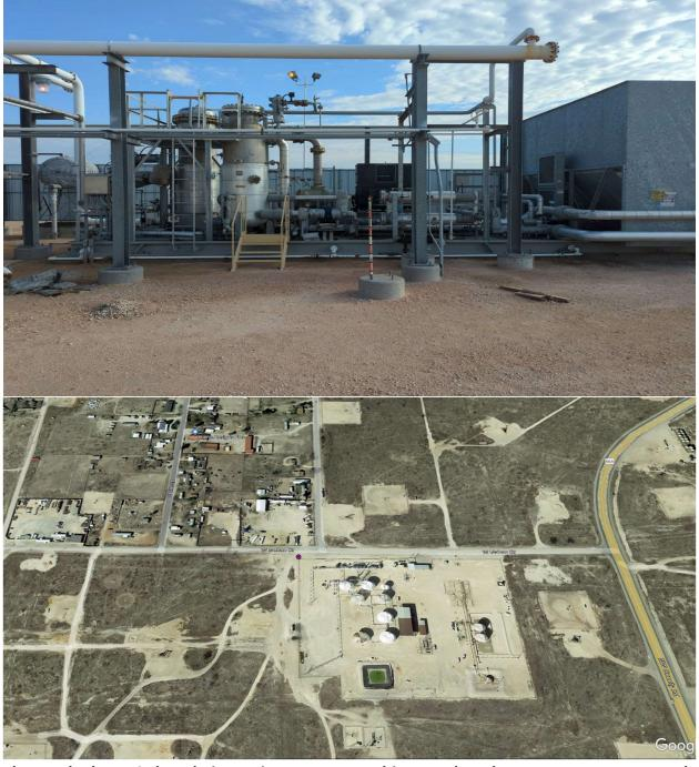
The North Plant RCF lost their F-train compressor. This caused our battery to pressure up and our Toromont compressor could not keep up and went down on HIHI discharge pressure The plant was having trouble getting their train back online so we had to begin shutting in wells in order to bring the inlet pressure down far enough for our compressor to run
