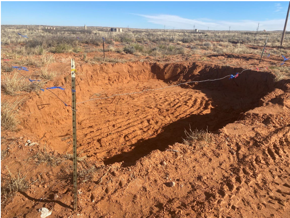
View of Area D excavation facing northeast.
