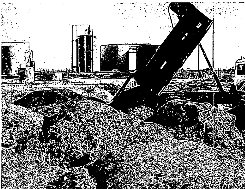
Backfilling with clean material
