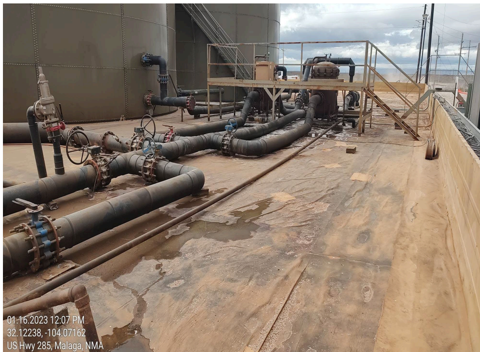
PHOTO 6: Containment Liner SW
