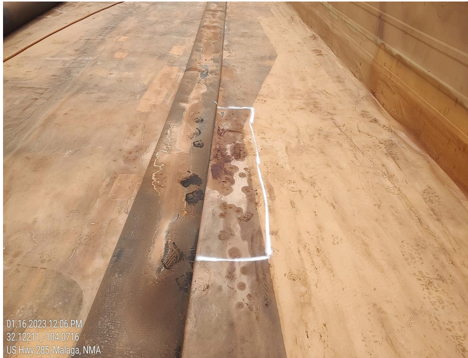
PHOTO 5: Cracks in Liner (Not Through Liner) Middle NE Side
