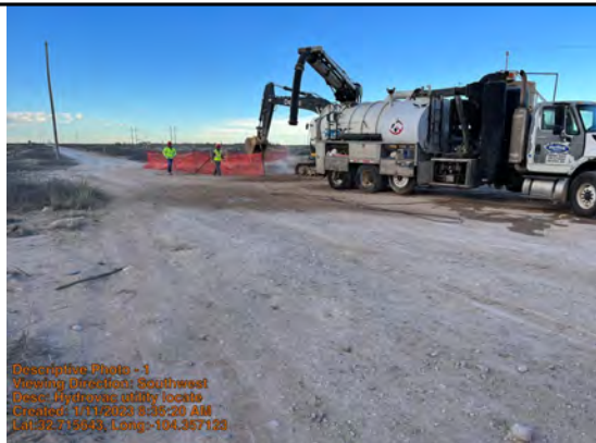
Hydrovac utility locate
