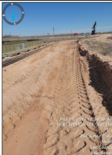
Photograph 4 Date: 03/29/2023 Description: Photo of excavation extent.
