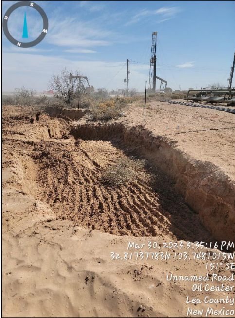
Photograph 5 Date: 03/30/2023 De: Photo of excavation.
