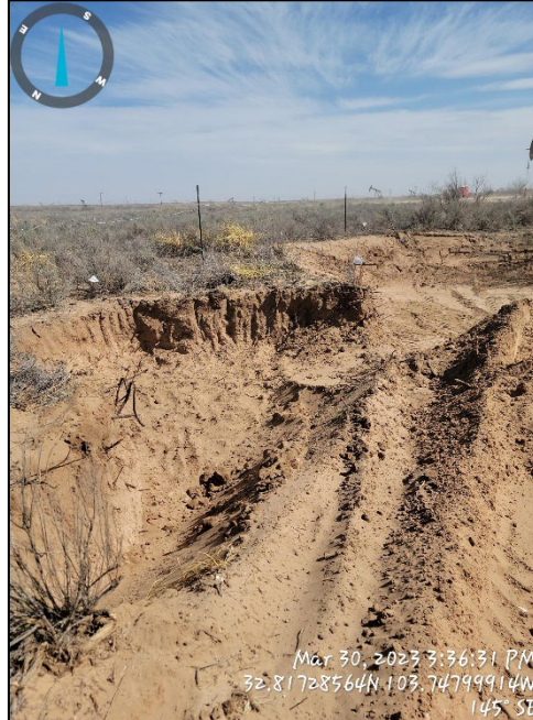
Photograph 6 Date: 03/30/2023 Description: Photo of excavation activities.
