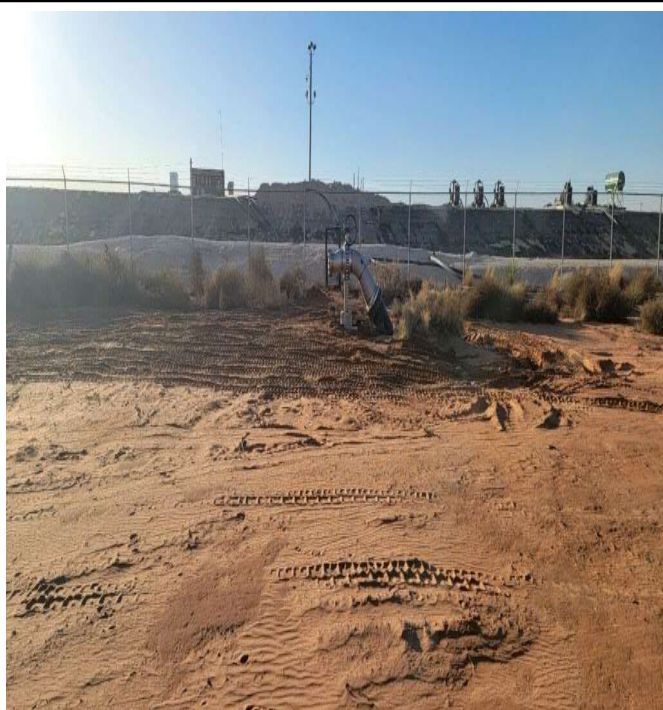
Backfilled to Grade
