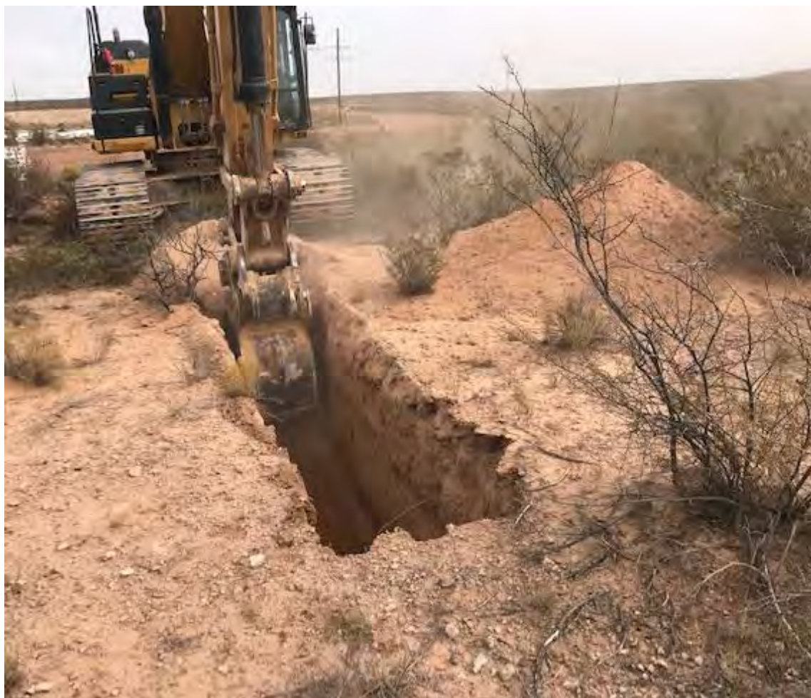
View of track-mounted backhoe advancing pothole PH16 during background soil sampling activities.
