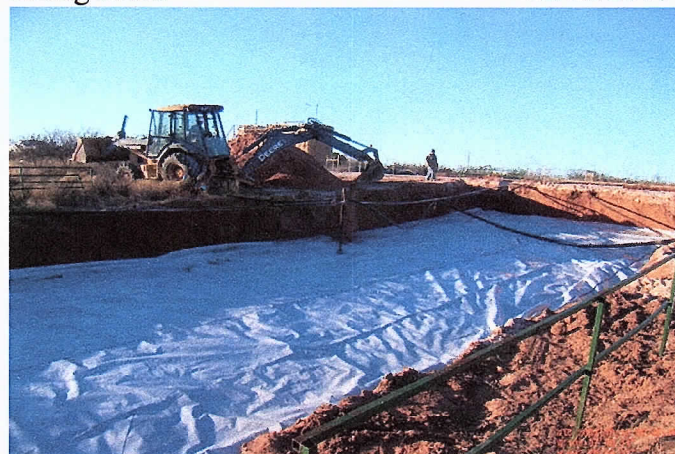
Padding the 20-mil, reinforced liner with imported soil, facing northeast
