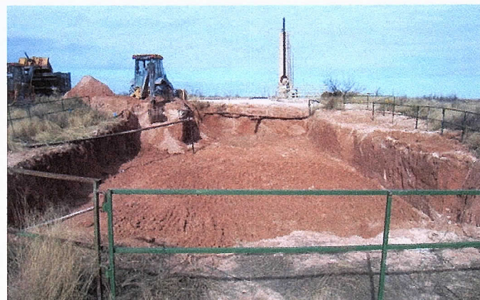
Excavating the site to 5 ft bgs, facing north
