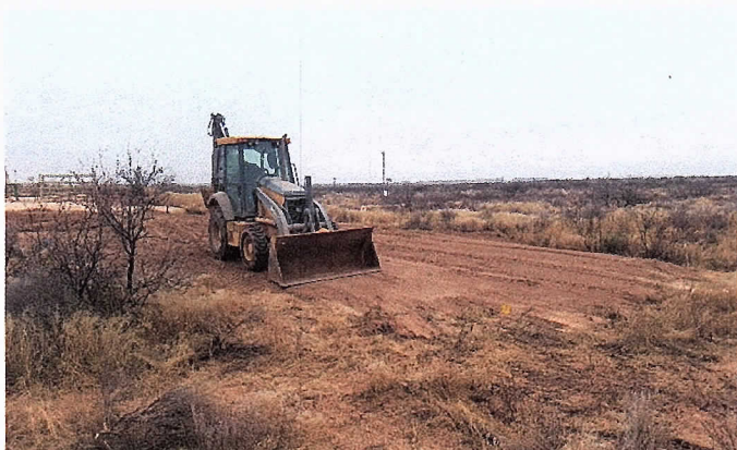
Backfilling and contouring the site with imported soil, facing west 12/27/2017
