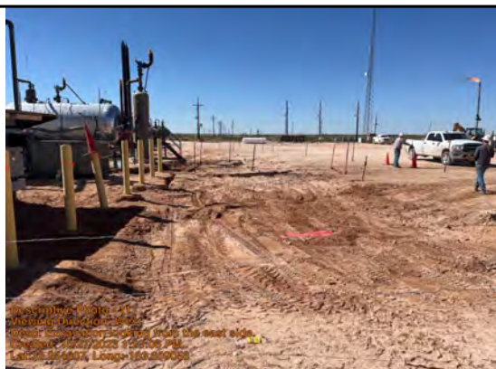
Excavation looking from the east side.
