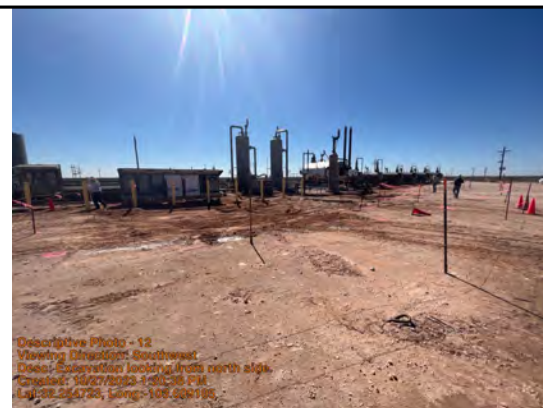
Excavation looking from north side.
