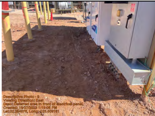
Deferred area in front of electrical panel.
