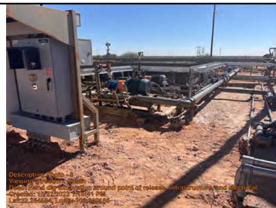
Viewing Direction: South
