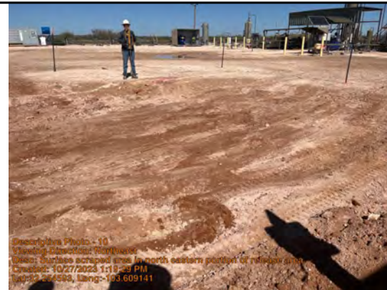
Surface scraped area in north eastern portion of release area.
