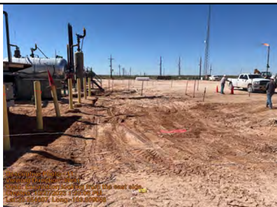
Excavation looking from the east side.
