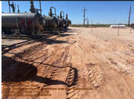
Viewing Direction: West
