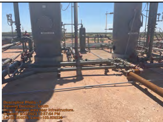
Viewing Direction: South
