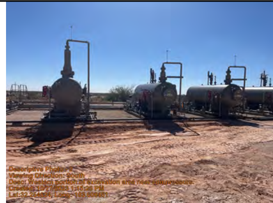
Viewing Direction: South
