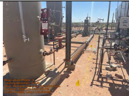
Viewing Direction: South
