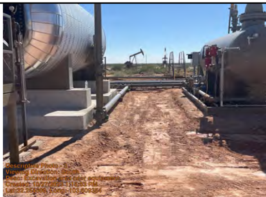
Viewing Direction: South
