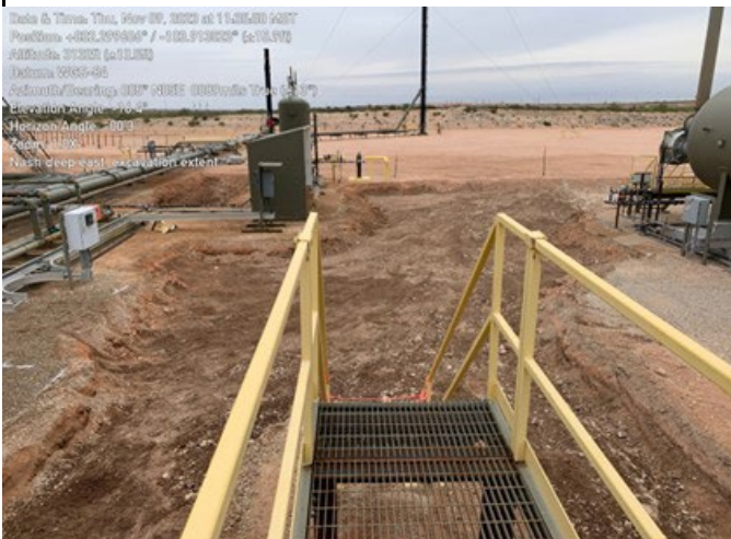
Photograph 3 Date: 11/09/2023 Description: Final excavation extent. View: North
