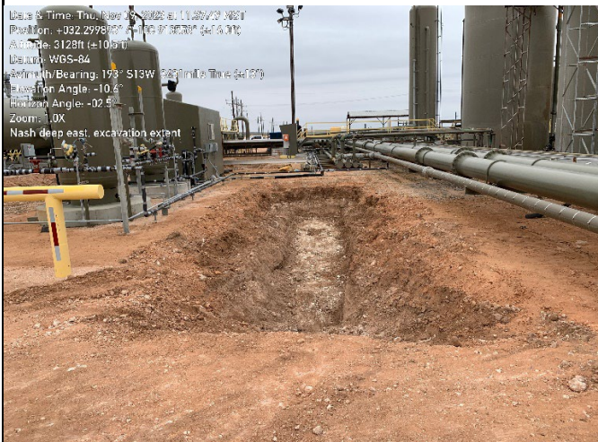
Photograph 4 Date: 11/09/2023 Description: Final excavation extent. View: South
