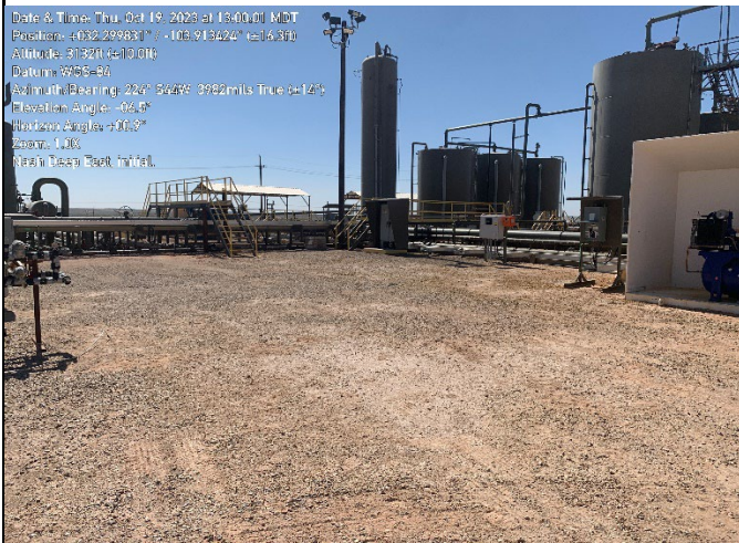
Photograph 1 Date: 10/19/2023 Description: Site assessment activities, release area. View: Southwest
