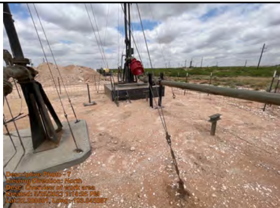
Overview of work area
