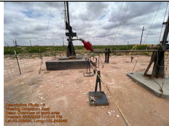
Overview of work area
