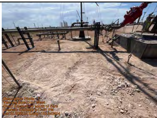
Excavation south of flare
