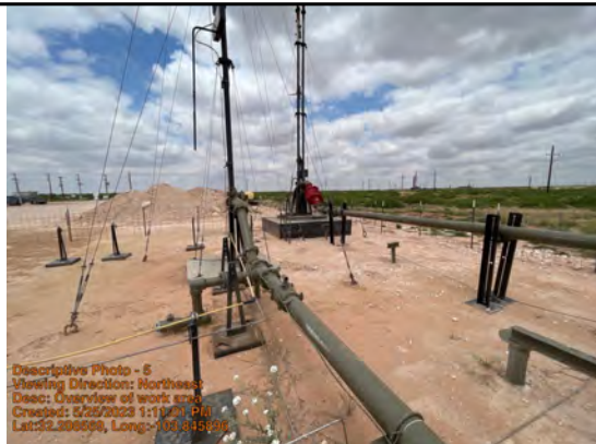
Overview of work area
