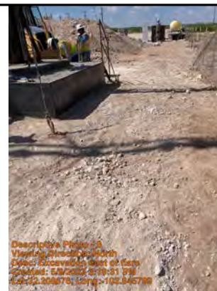
Excavation east of flare
