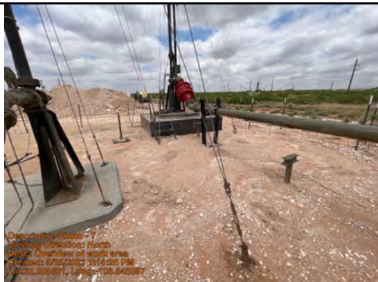
Overview of work area
