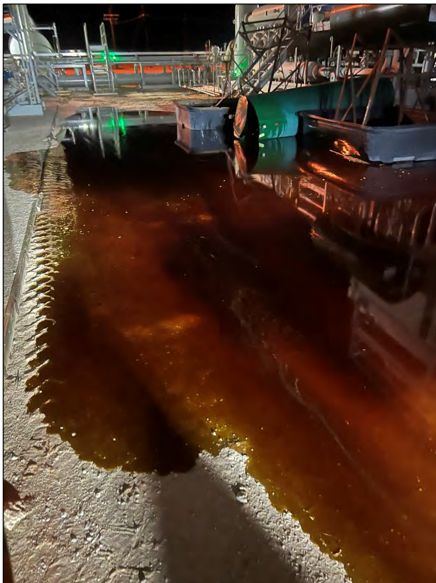
Photo 1. Lube oil release at time of discovery.
