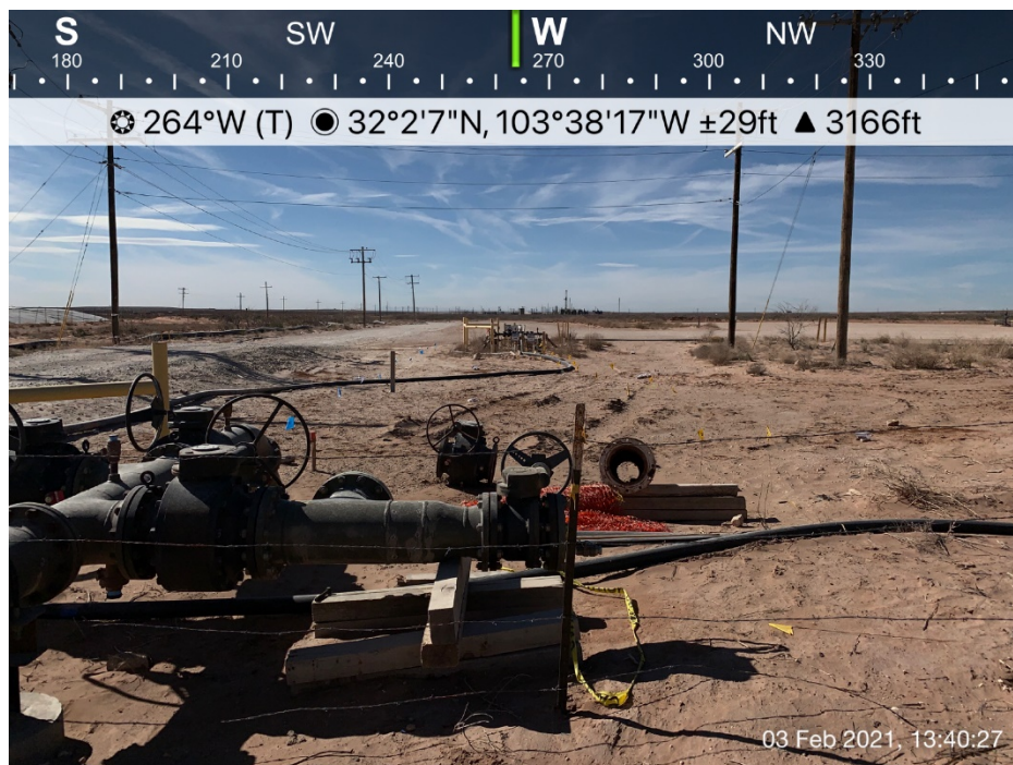
Impacted area viewing West, February 3, 2021
