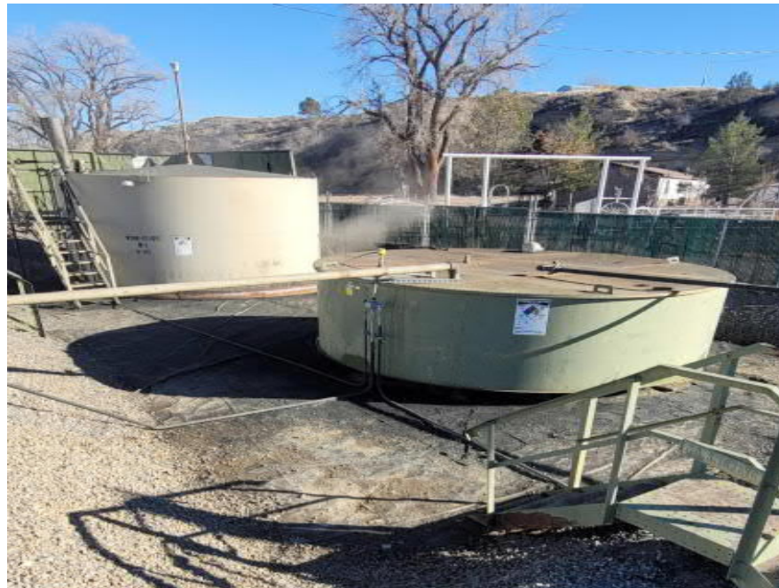
Photograph 2 (dated 12/6/2023) – View looking SE at secondary containment with the liner exposed.
