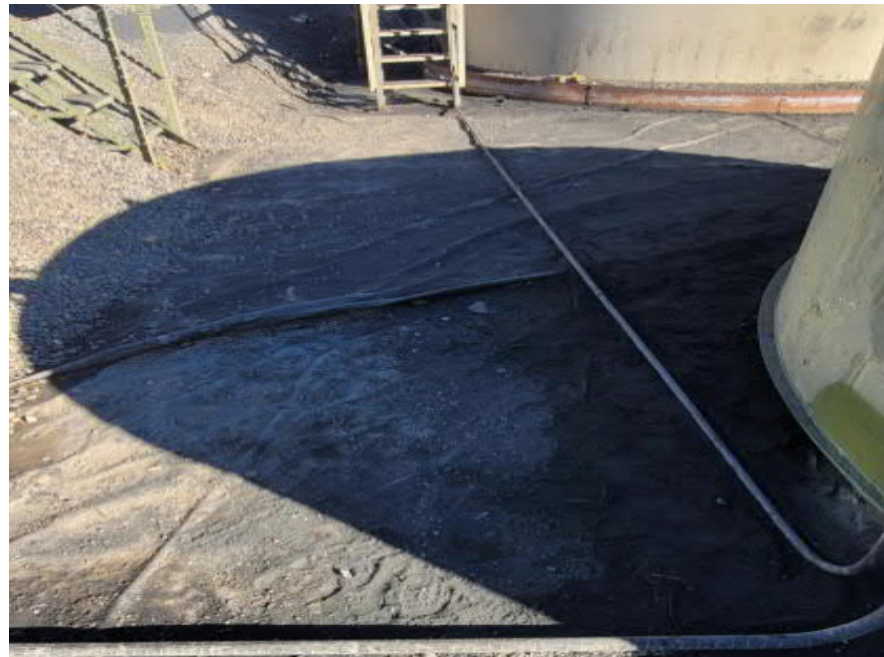
Photograph 4 (dated 12/6/2023) – View looking E at the exposed liner between the storage tank and pit tank.
