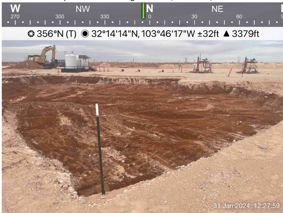
Additional excavated area viewing north, January 31, 2024
