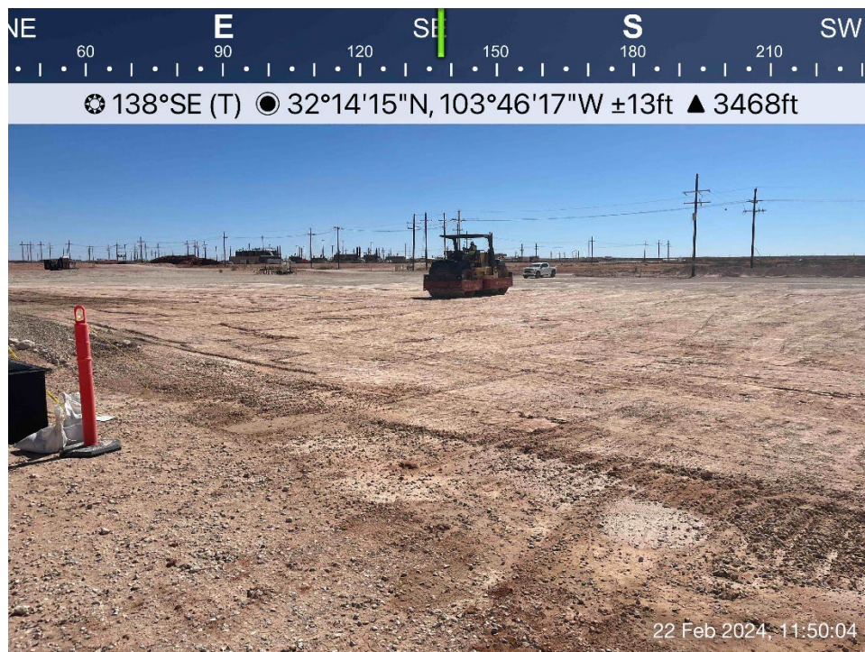
Backfilled and rolled excavated area viewing southeast, February 22, 2024
