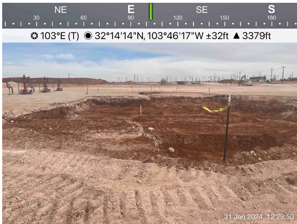
Additional excavated area viewing east, January 31, 2024
