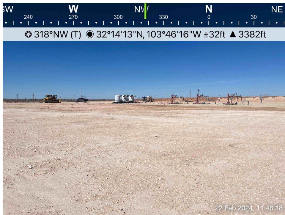
Backfilled and rolled excavated area viewing northwest, February 22, 2024
