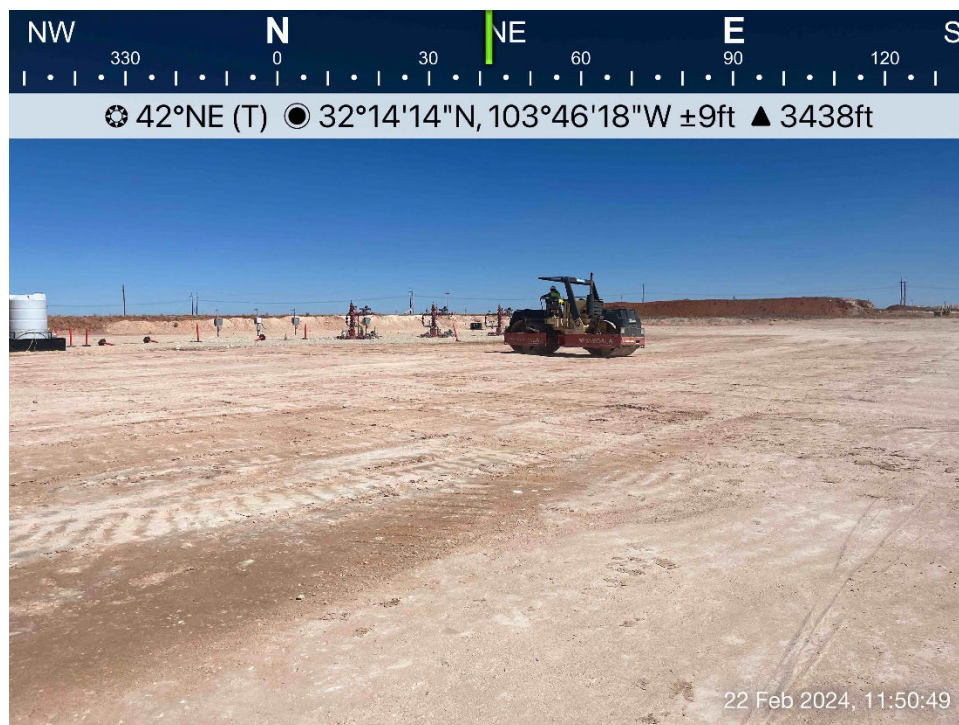
Backfilled and rolled excavated area viewing northeast, February 22, 2024
