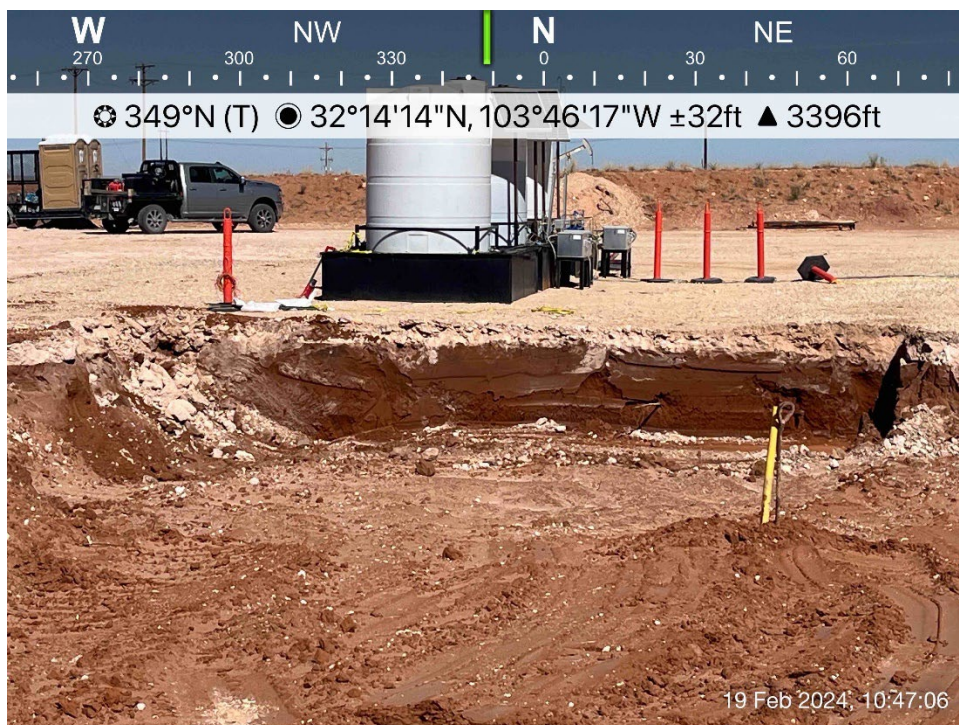
Additional excavated area viewing north, February 19, 2024
