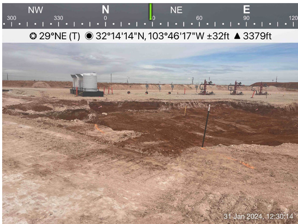
Additional excavated area viewing northeast, January 31, 2024
