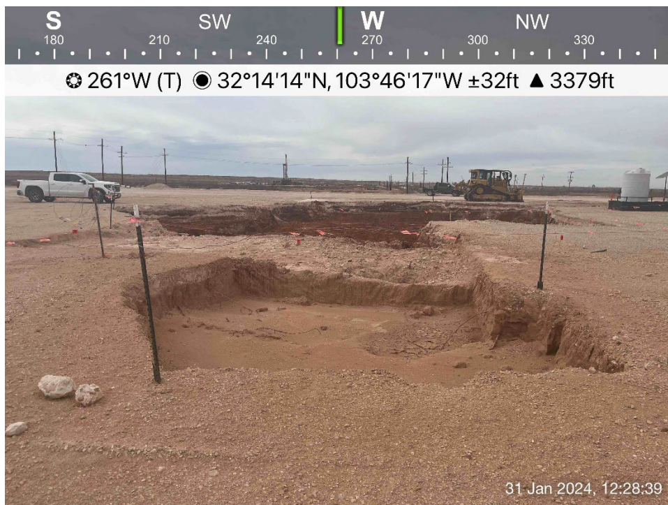
Additional excavated area viewing west, January 31, 2024
