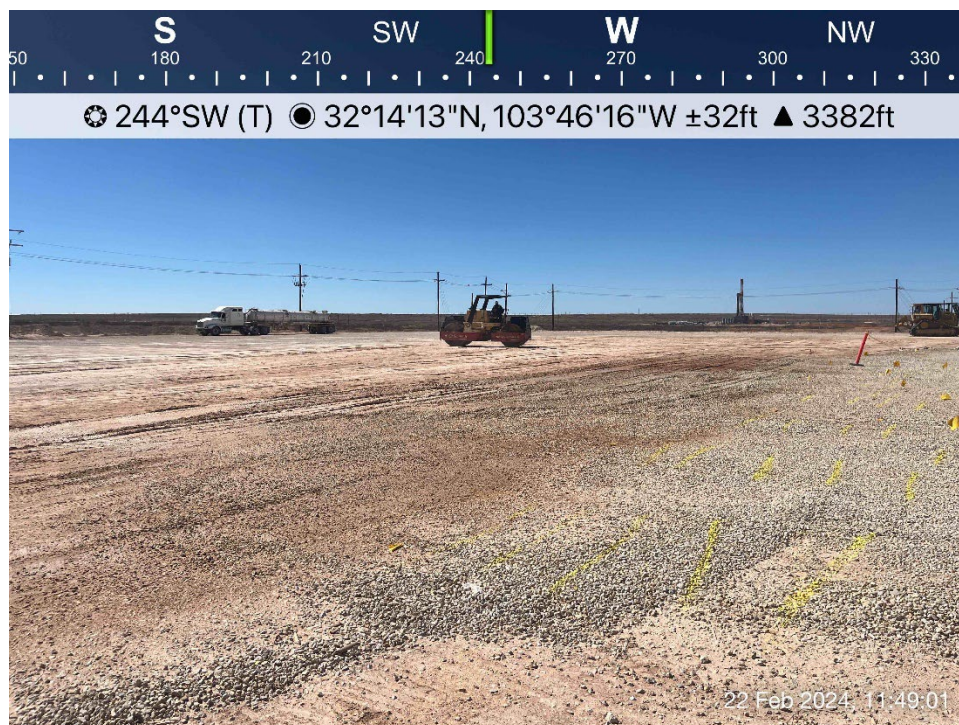
Backfilled and rolled excavated area viewing southwest, February 22, 2024
