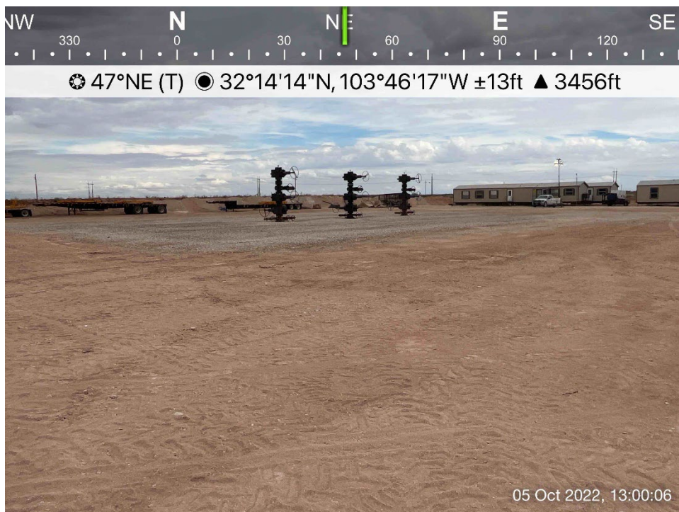
Impacted area viewing southwest, October 5, 2022
