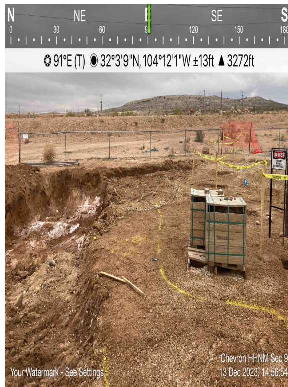
View of Remediation – View East
