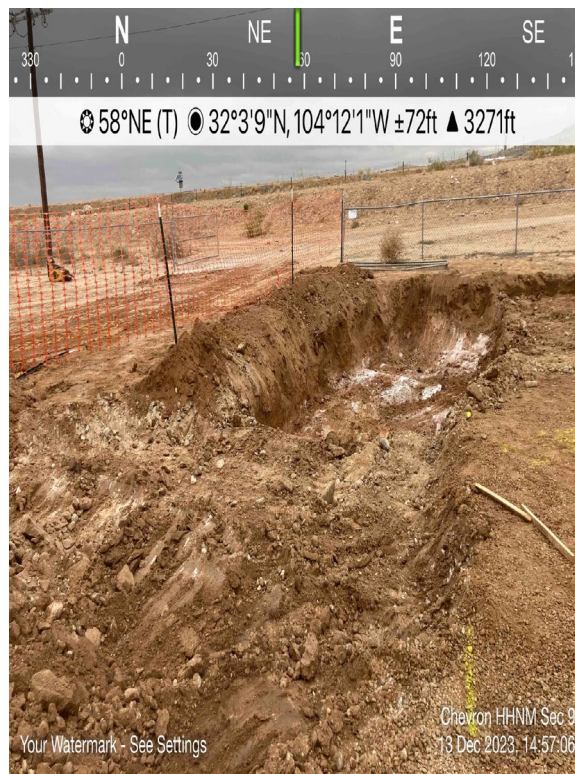
View of Remediation – View Northeast
