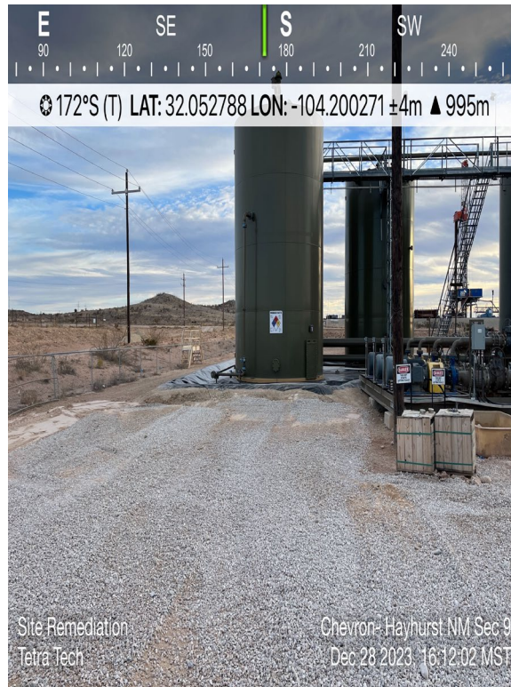
View of Backfilled Area – View South
