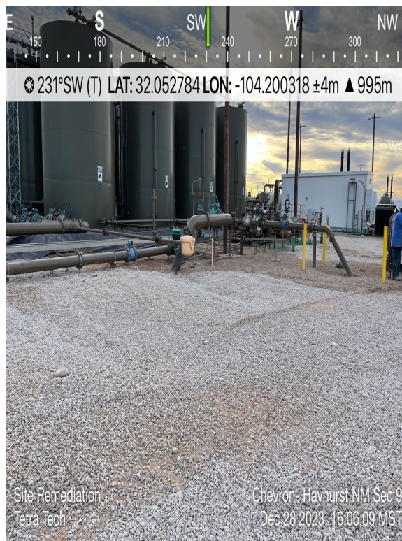
View of Backfilled Area – View Southwest
