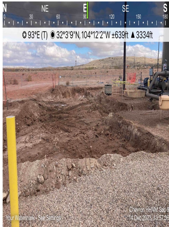
View of Remediation – View East
