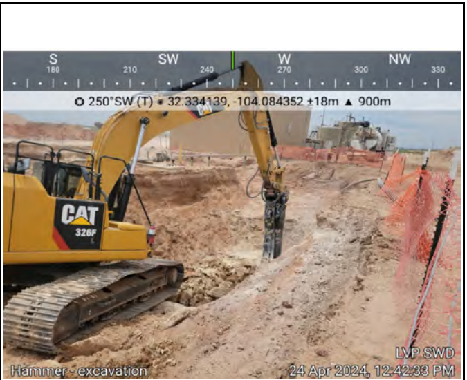
Photograph: 2 Date: 4/18/24 Description: Excavation through conglomerate soil View: North
