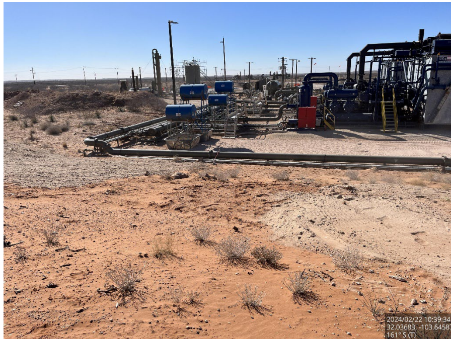
Backfilled and seeded excavation in pasture, viewing to the south.
