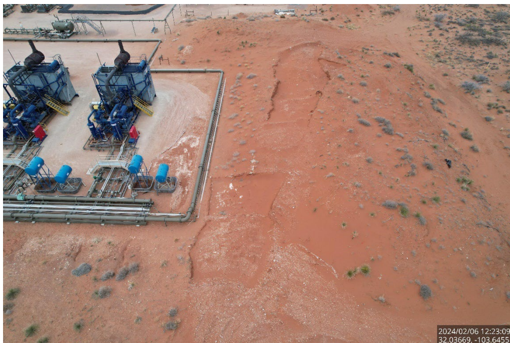
Aerial image of the excavation, viewing to the west.
