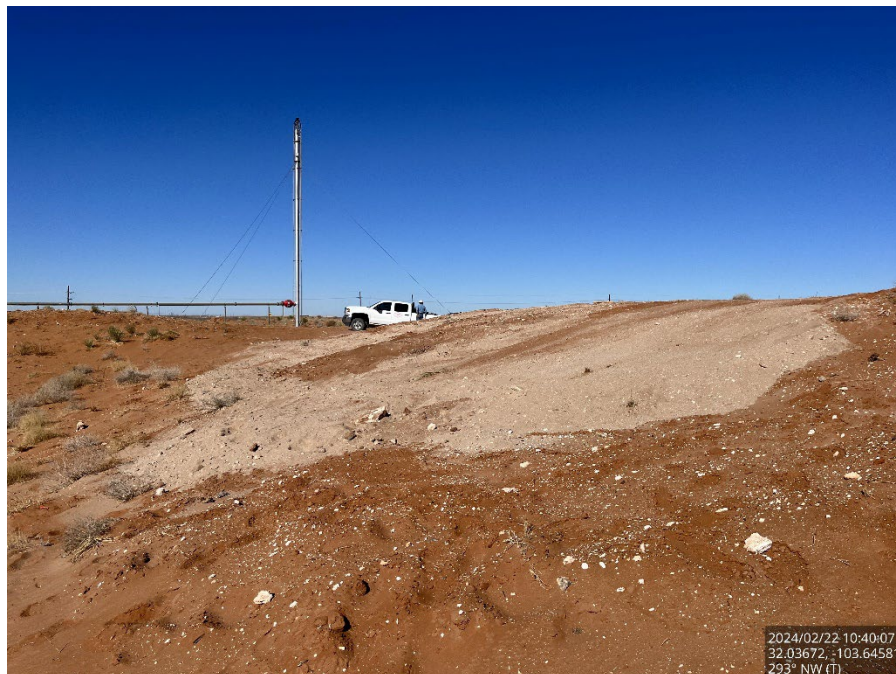
Backfilled and seeded excavation in pasture, viewing to the northwest.
