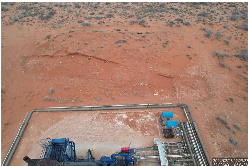
Aerial image of the excavation, viewing to the north.
