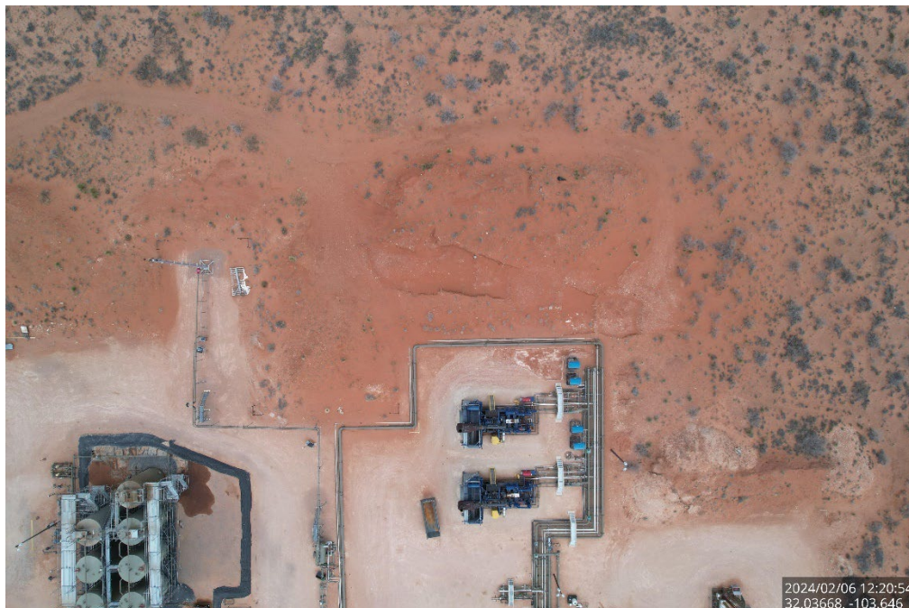
Aerial image of the excavation, vertical view.
