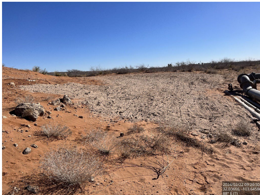
Backfilled and seeded excavation in pasture in pasture, viewing to the east.
