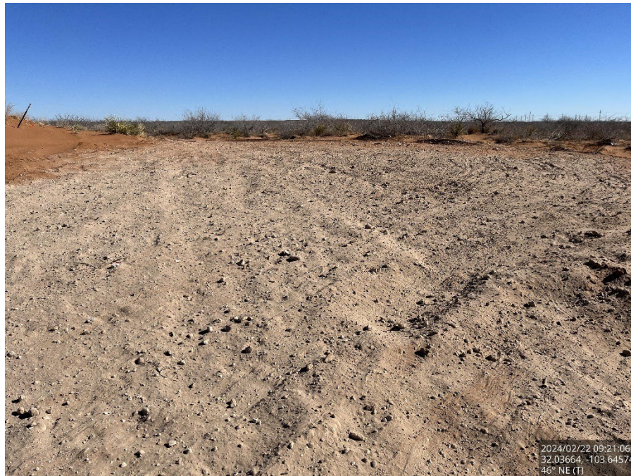
Backfilled and seeded excavation in pasture, viewing to the northeast.
