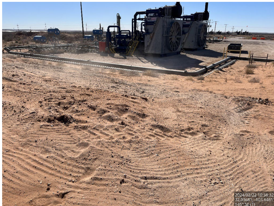
Backfilled and seeded excavation in pasture, viewing to the southeast.
