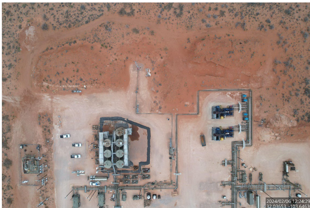
Aerial image of the excavation, vertical view.
