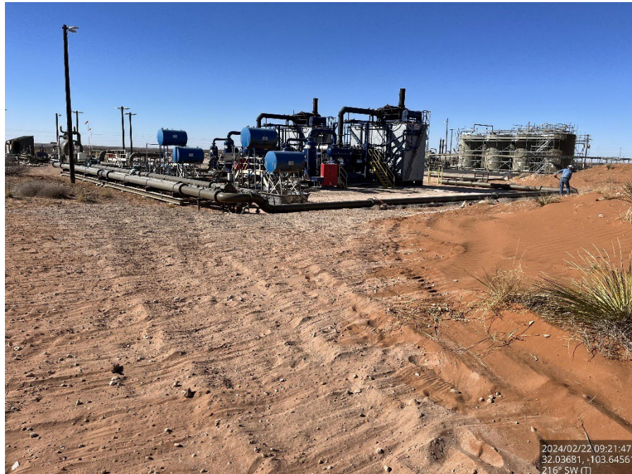
Backfilled and seeded excavation in pasture, viewing to the southwest.
