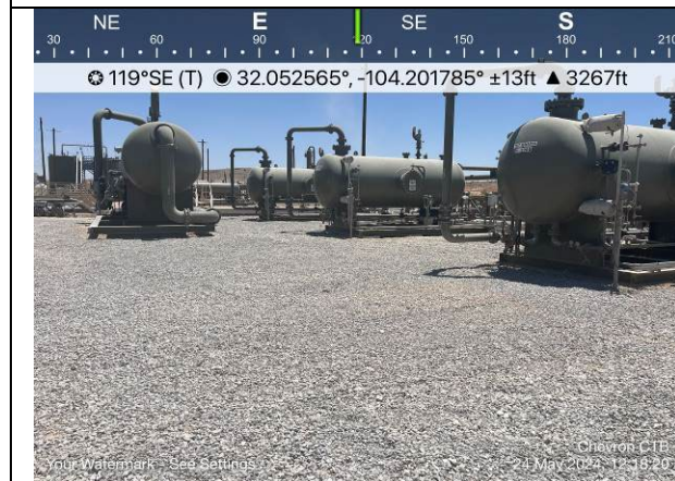
Photo 9: View of backfilled Site post-remediation.
