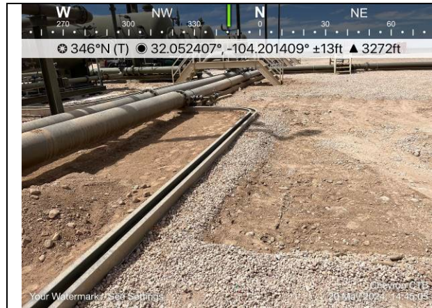
Photo 7: View of remediation activities.
