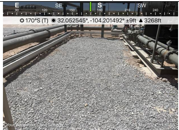
Photo 10: View of backfilled Site post-remediation.
