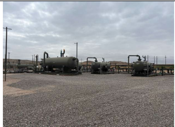
Photo 8: View of backfilled Site post-remediation.
