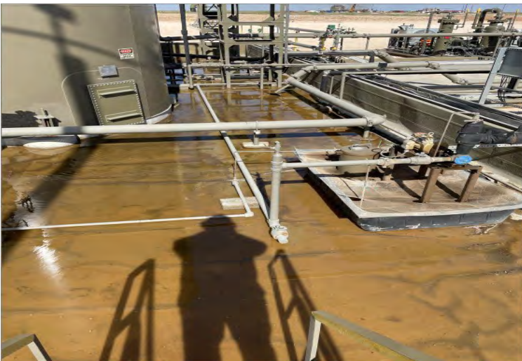
Released Fluid in Containment
