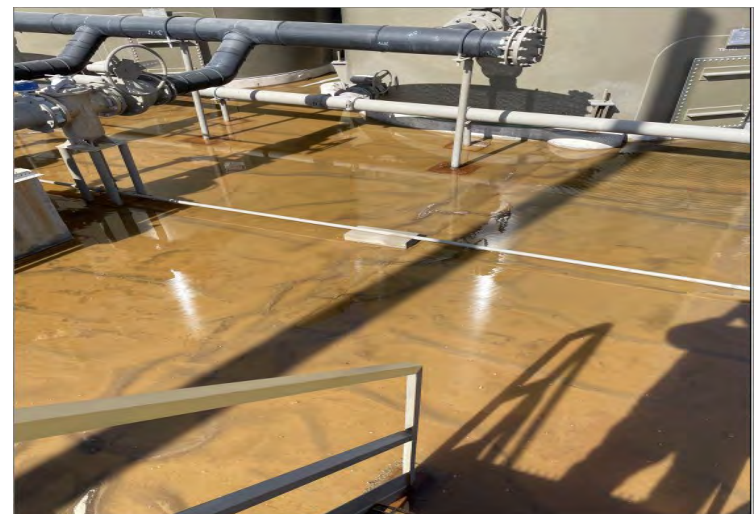
Release Fluid in Containment
