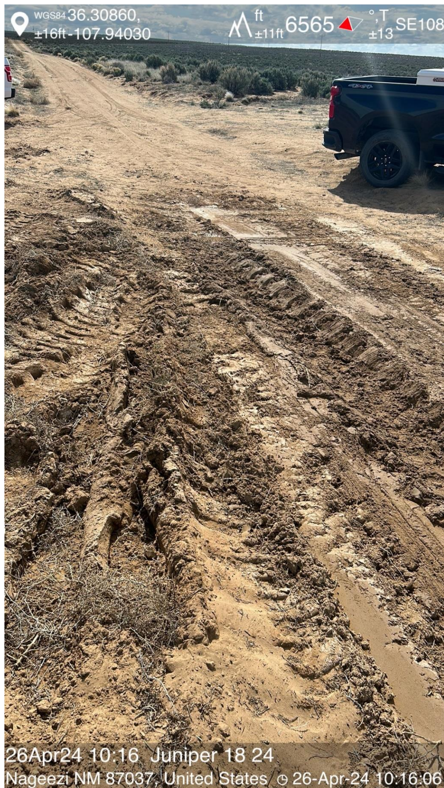
Spill flow area at the Juniper 18-24 showing where produced water flowed and collected on well location access road.
