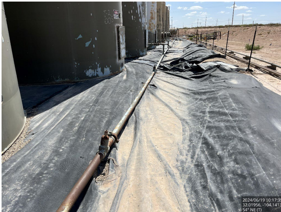
Lined tank battery containment where release occurred, viewing to the northeast.
