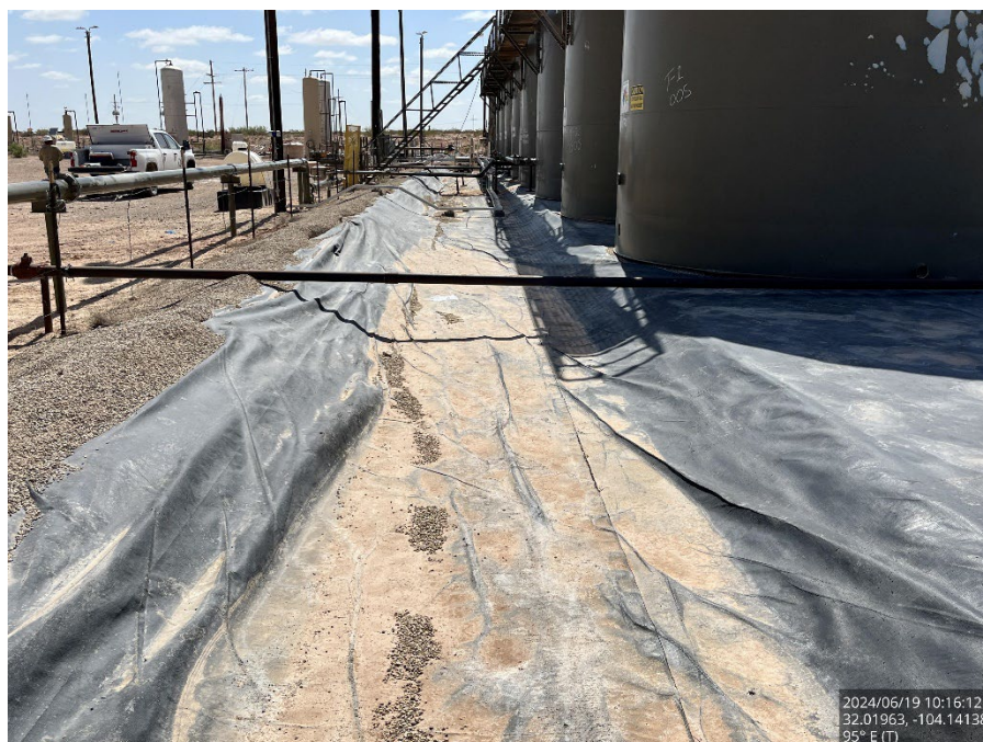
Lined tank battery containment where release occurred, viewing to the east.
