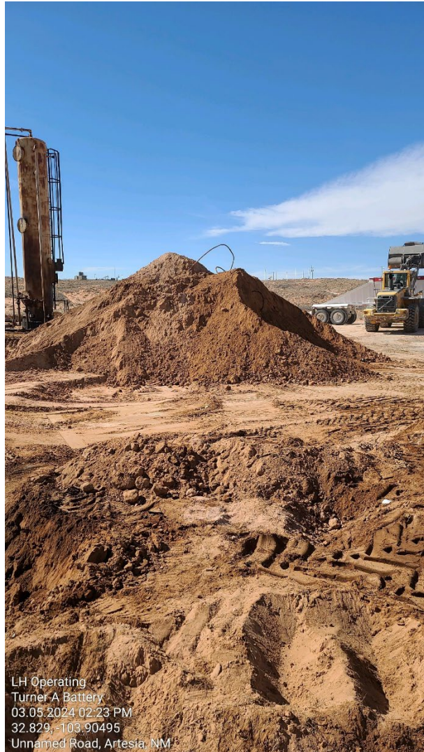
Turner A Battery (nAPP2403039770)
