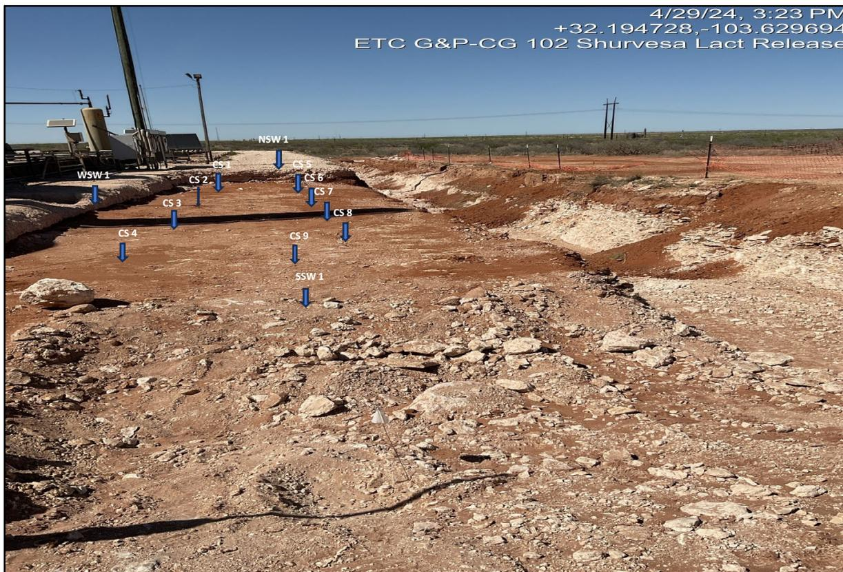
View North - Remediation activities (i.e., excavation and stockpiling) and sampling CS 1 thru CS 9, WSW 1, NSW 1 and SSW 1 in progress. Date: Apr 29, 2024
