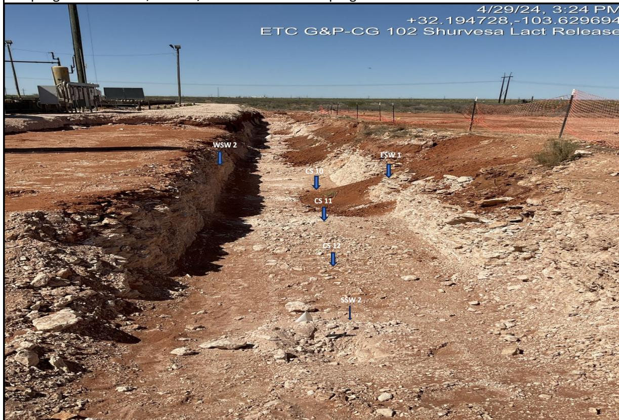
View North - Remediation activities (i.e., excavation and stockpiling) and sampling CS 10 thru CS 12, WSW 2, ESW 1 and SSW 2 in progress. Date: Apr 08, 2024
