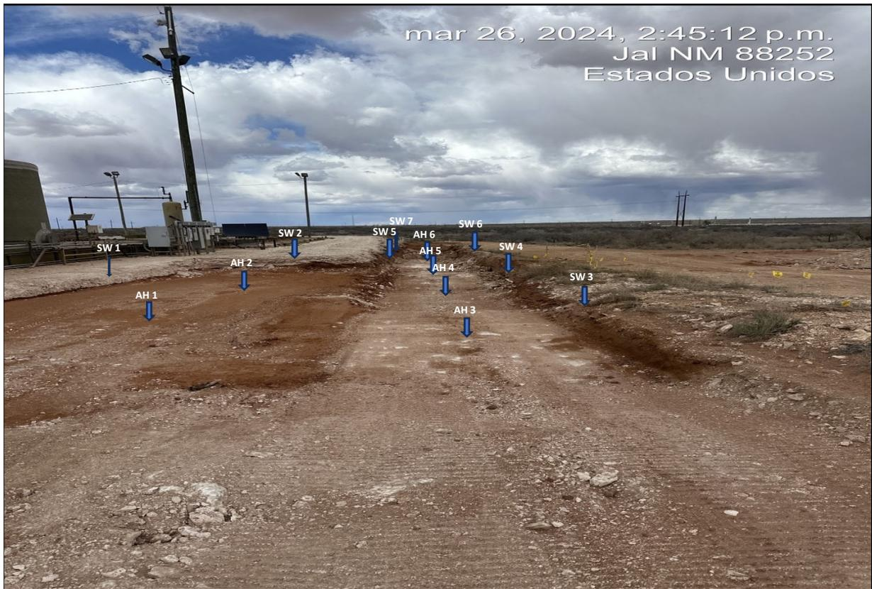
View North - Remediation activities (i.e., excavation and stockpiling) and sampling of AH 1 thru AH 6 and SW 1 thru SW 7 in progress. Date: Mar 26, 2024
