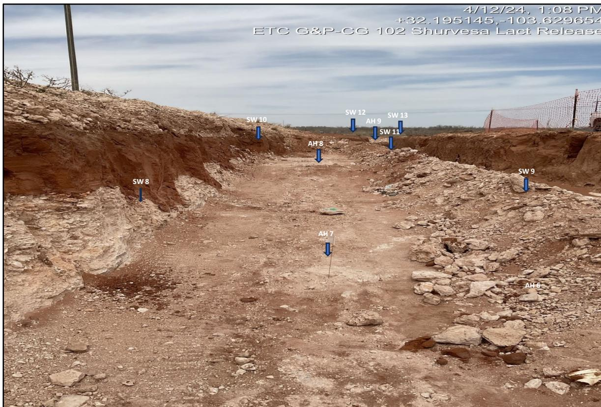
View North - Remediation activities (i.e., excavation and stockpiling) and sampling of AH 7 thru AH 9 and SW 8 thru SW 13 in progress. Date: Apr 12, 2024
