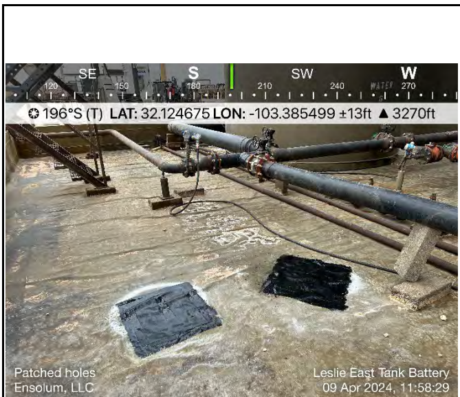
Photograph 6 Description: Liner inspection View: East
