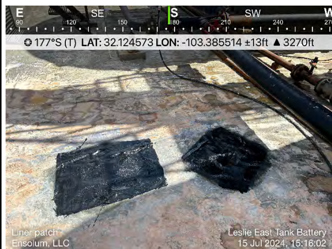
Photograph 12 Description: Repair liner View: South
