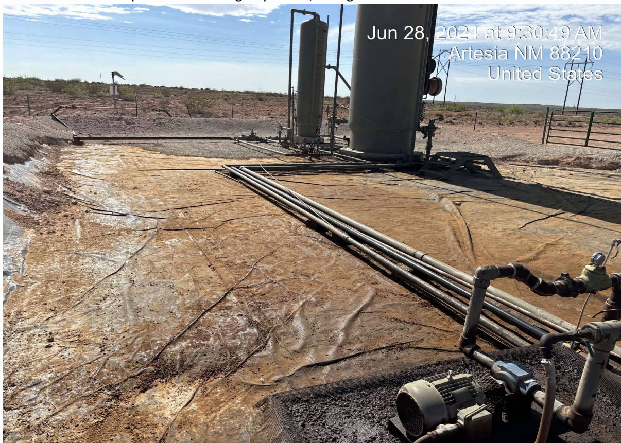
Photo 4 - View of exposed liner during inspection, facing Southeast.
