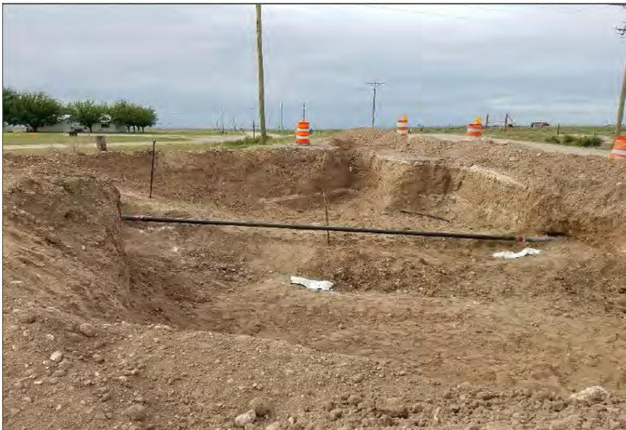
Excavated area before placing liner looking to south
