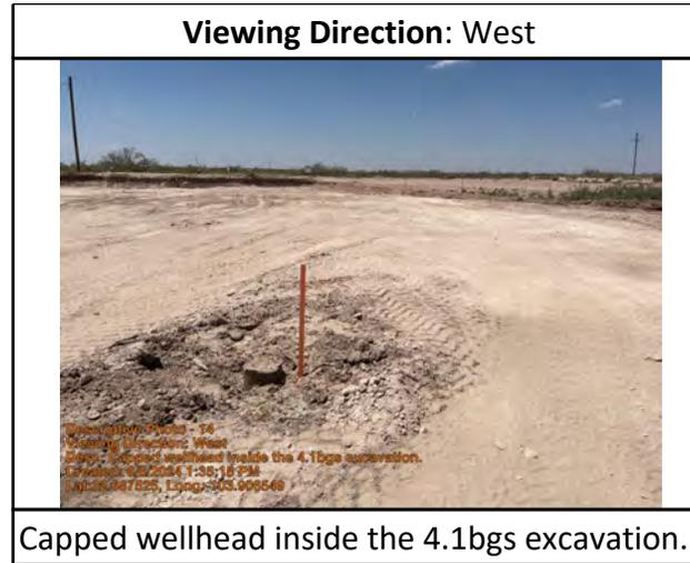
Capped wellhead inside the 4.1ft bgs excavation.
