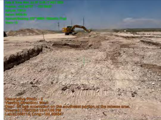
3ft bgs excavation on the southeast portion of the release area.
