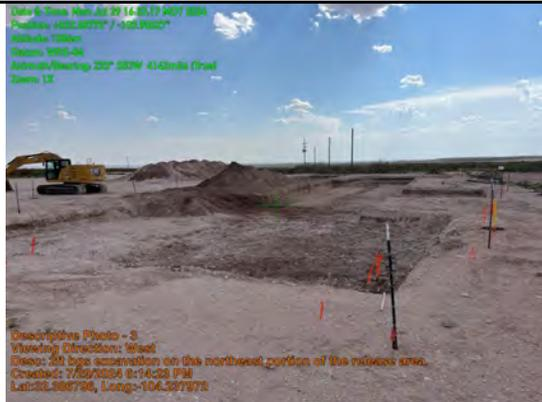
2ft bgs excavation on the northeast portion of the release area.
