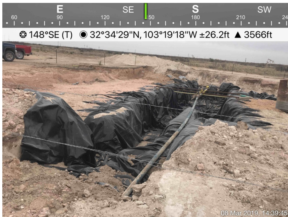
Lined Excavation Prior to Cutting and Purging the Flowline, March 8, 2019
