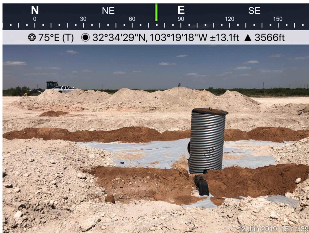
Sand Padding over Flowlines Viewing East, June 12, 2019
