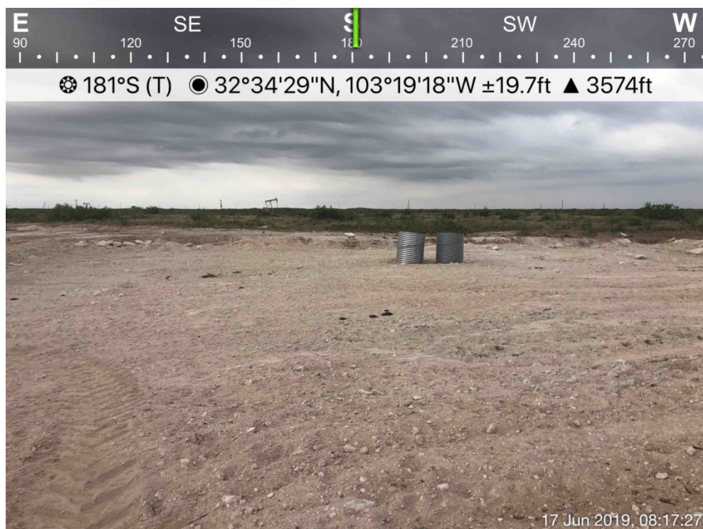
Caliche Filled Excavation to 1.5 feet bgs Viewing South, June 17, 2019
