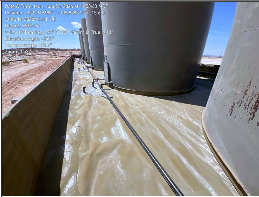
PHOTO 5: Southwest view of the lined secondary containment during liner inspection. 08/26/2024
