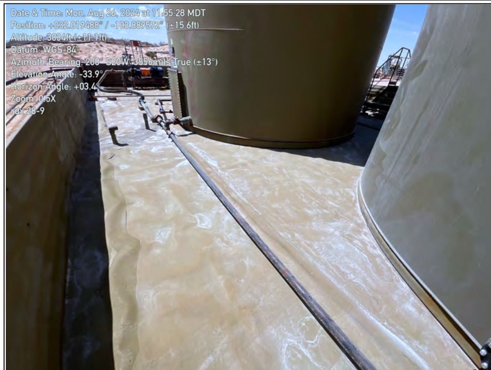
PHOTO 8: Southwest view of the lined secondary containment during liner inspection. 08/26/2024
