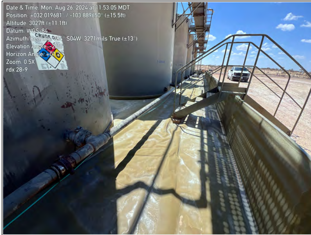
PHOTO 3: Southwest view of the lined secondary containment during liner inspection. 08/26/2024
