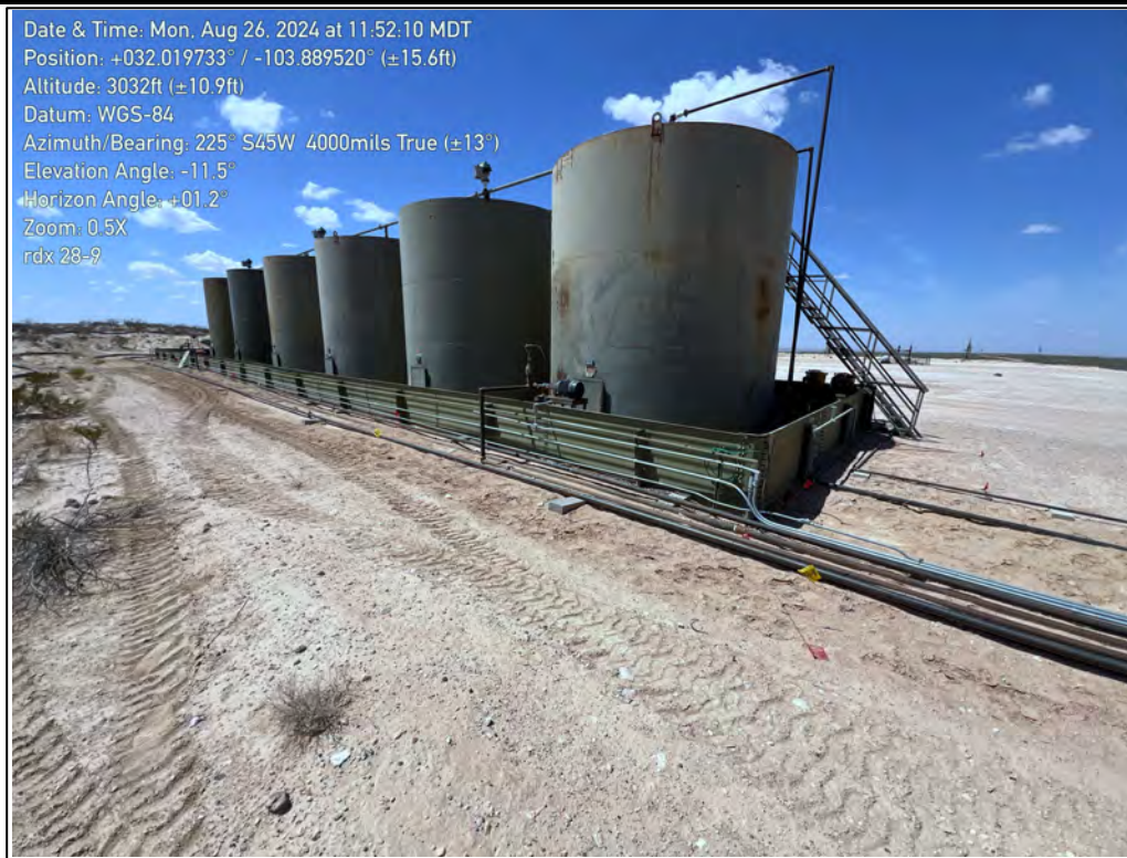
PHOTO 11: Southwest exterior view of the lined secondary containment during liner inspection. 08/26/2024
