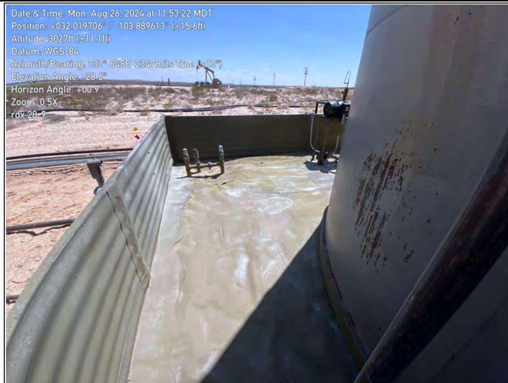
PHOTO 4: Southeast view of the lined secondary containment during liner inspection. 08/26/2024
