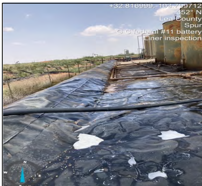
Photo exposing liner pursuant to gravel removal, taken facing Northwest.
