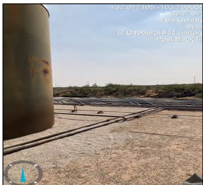
Photo of liner pursuant to backfill, taken facing Southwest.
