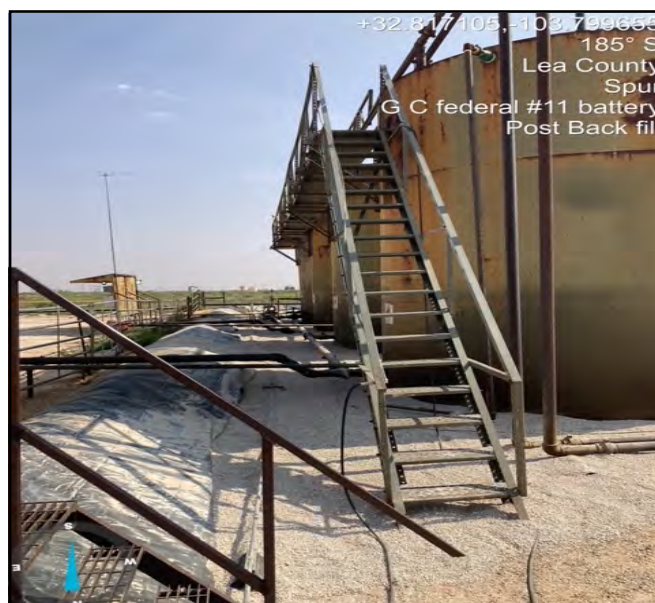
Photo of liner pursuant to backfill, taken facing South.
