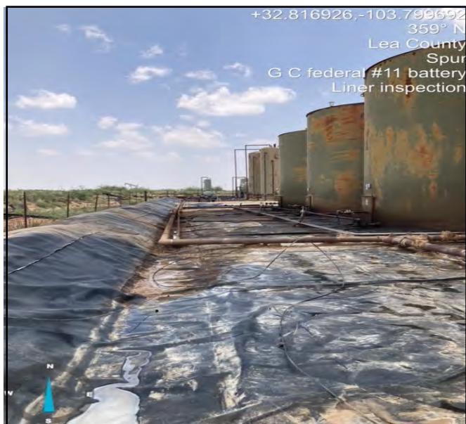
Photo exposing liner pursuant to gravel removal, taken facing North.
