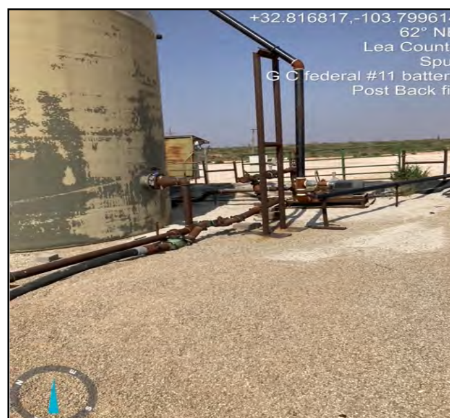
Photo of liner pursuant to backfill, taken facing Northeast.
