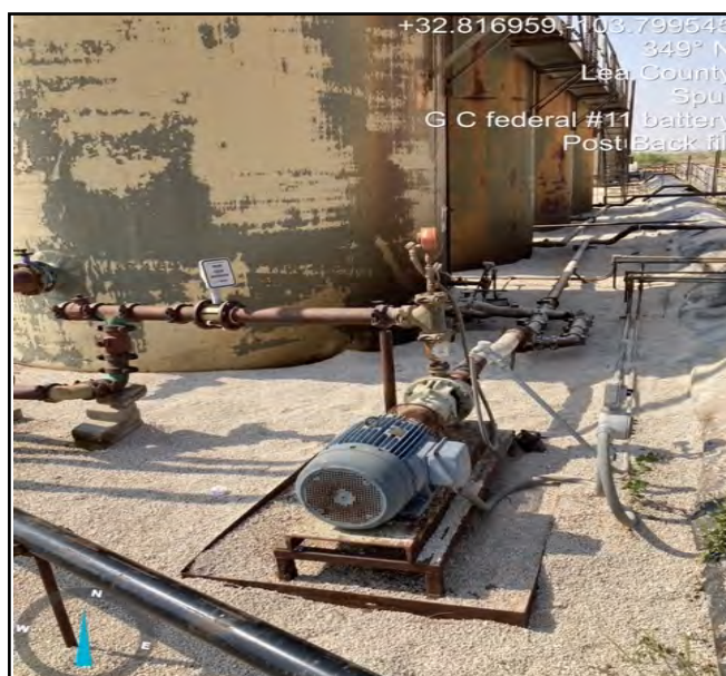
Photo of liner pursuant to backfill, taken facing Northwest.
