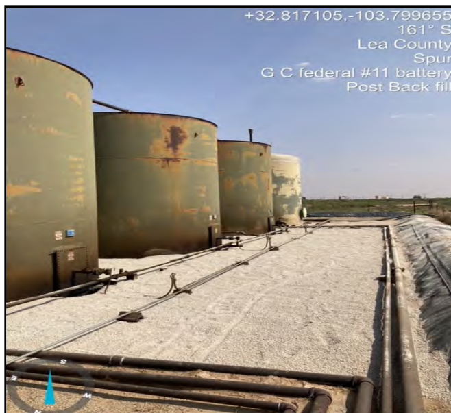
Photo of liner pursuant to backfill, taken facing Southeast.
