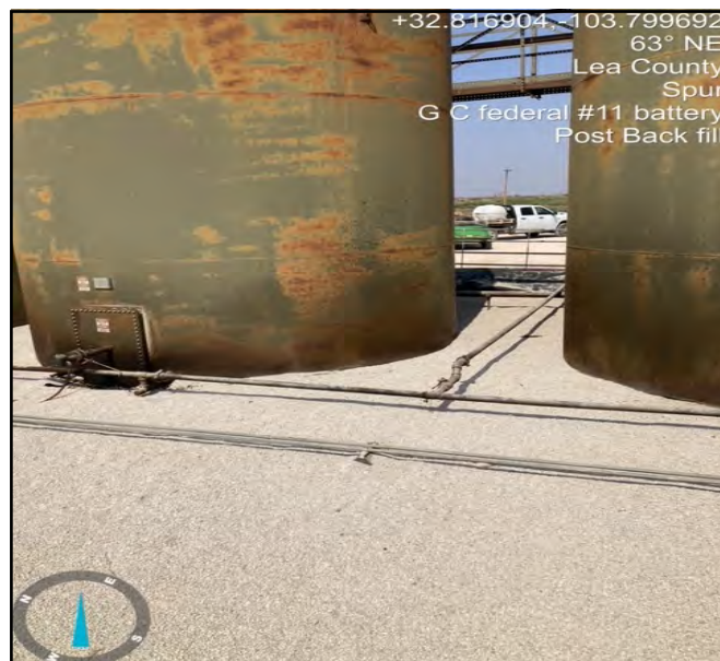
Photo of liner pursuant to backfill, taken facing Northeast.
