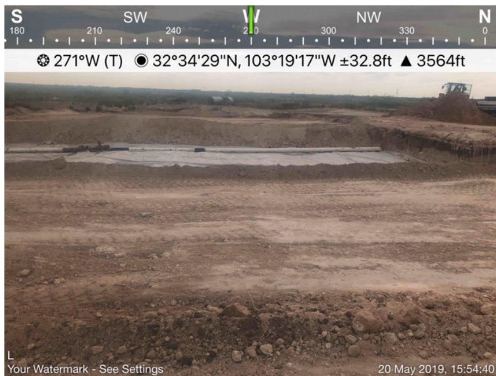
Excavation Backfilling Viewing West, May 20, 2019
