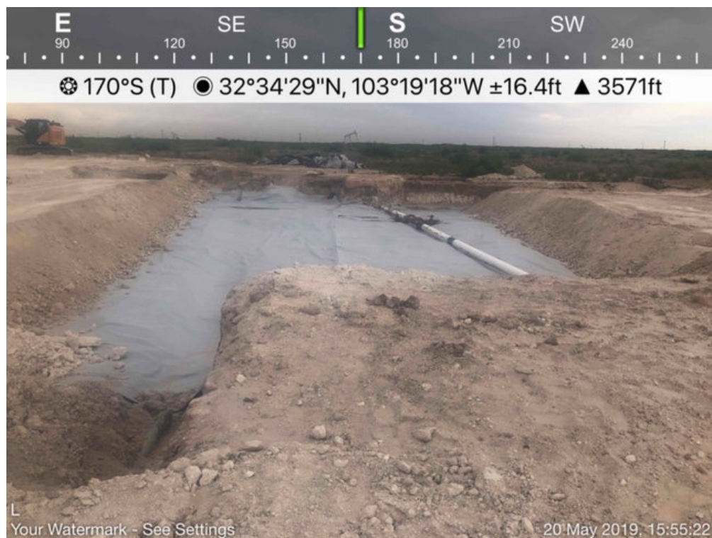
Excavation Backfilling Prior to Installing New Fiberglass Line Viewing South
