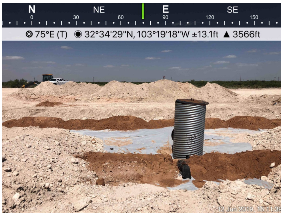
Sand Padding over Flowlines Viewing East, June 12, 2019
