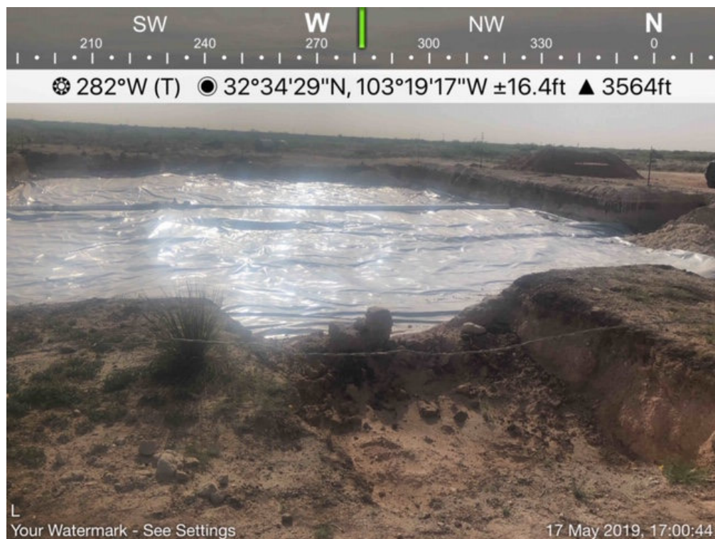
Liner Installation Viewing West, May 17, 2019
