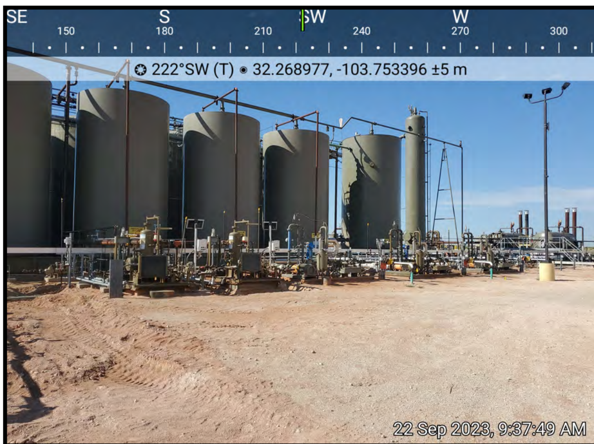
View of the excavated area, facing southwest.
