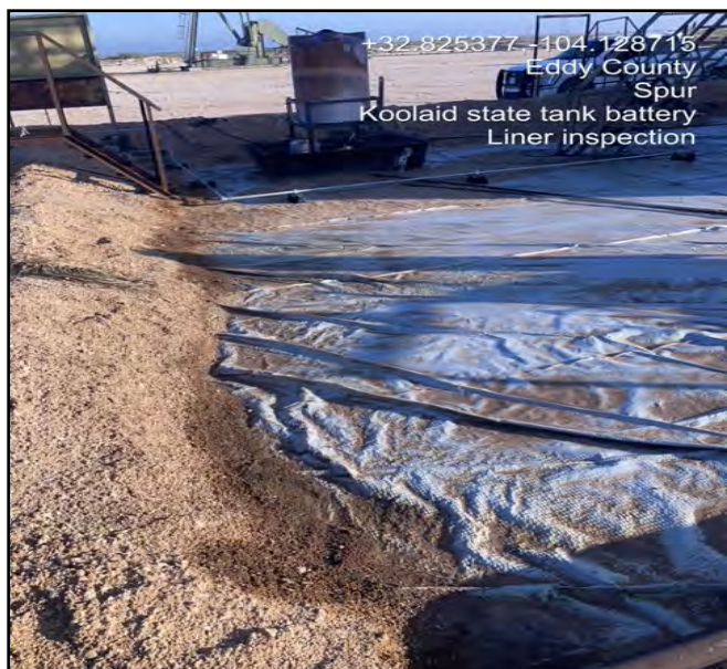
Image of liner pursuant to being power washed.
