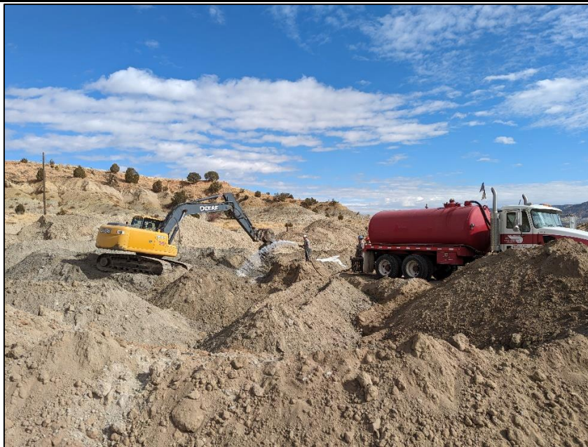
Photograph: 3 Date: 11/16/2023 Description: Applying Micro-Blaze amendment to soil removed from the excavation View: East
