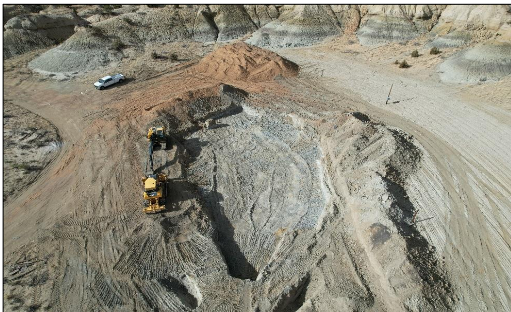
Photograph: 1 Date: 11/15/2022 Description: Excavation of impacted soil View: Aerial view looking west
