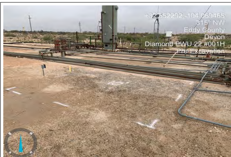
Flagging/marking excavation area
