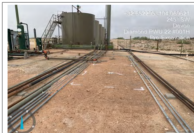
Flagging/marking excavation area
